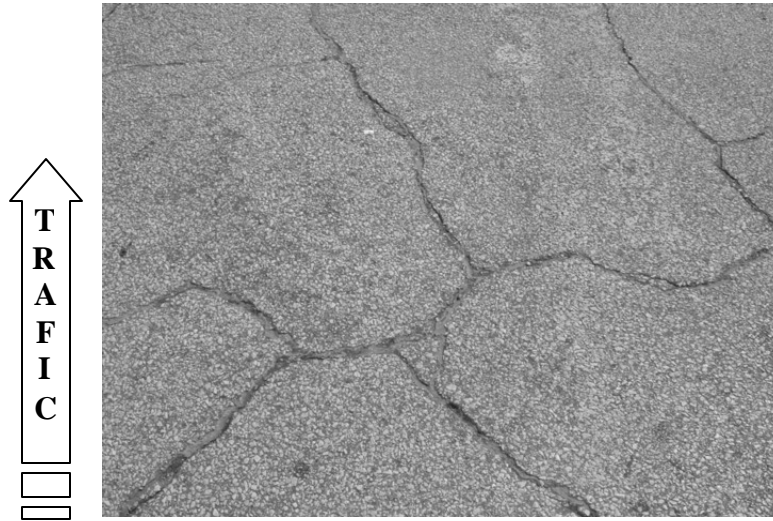
Figure 1.2 Block cracking
