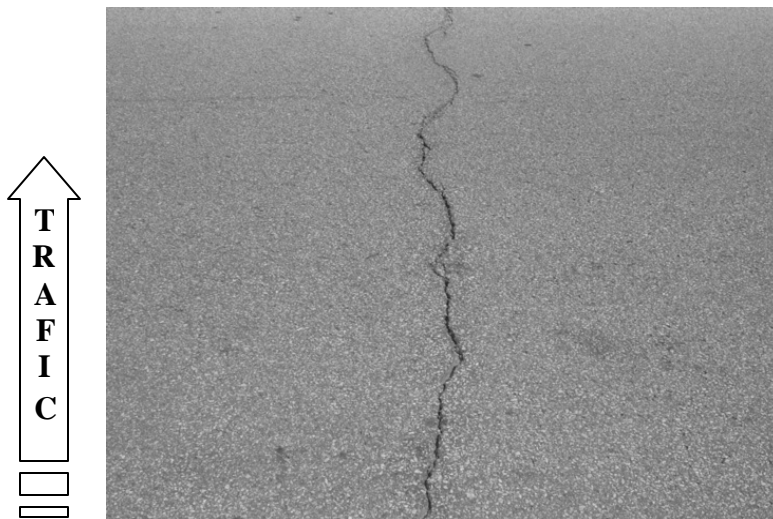
Figure 1.3 Longitudinal cracking
