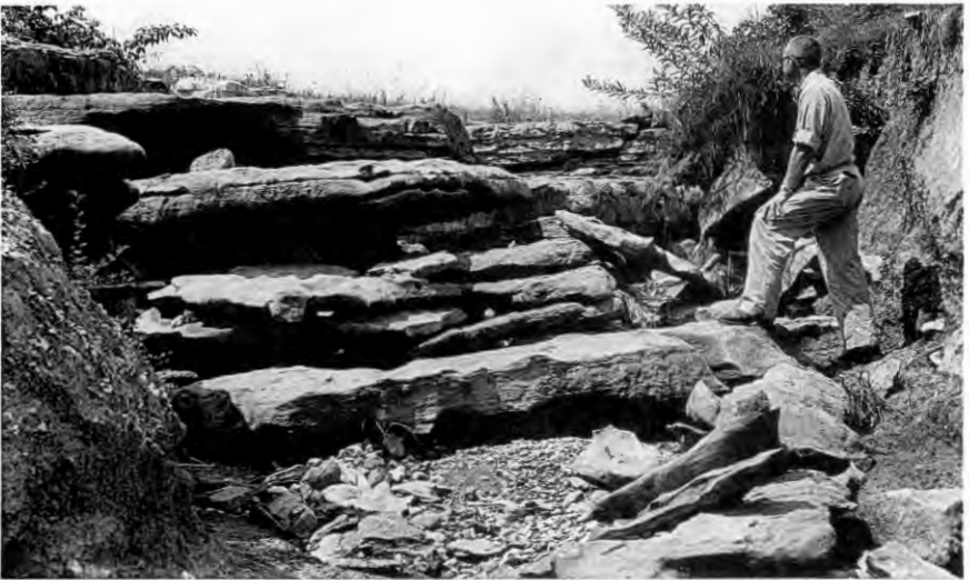
B. NORTH VERNON LIMESTONE IN SPILLWAY OF A SMALL RESERVOIR AT LOCATION 6 IN THE EAST-CENTRAL PART OF SEC. 22, T. 5 N., R. 8 E. EARTH FILL OF THE DAM IS AT RIGHT OF PHOTOGRAPH.
