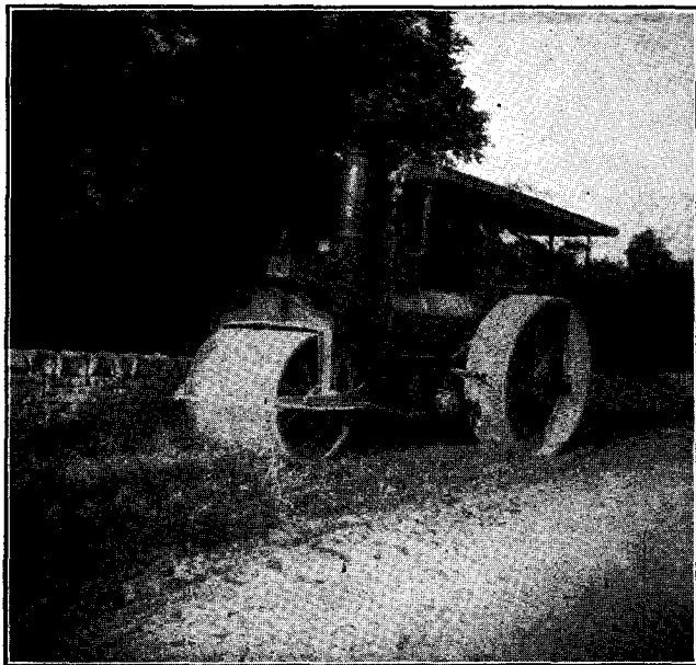
Steam road roller used in Bloomington. Weight 12 tons.
