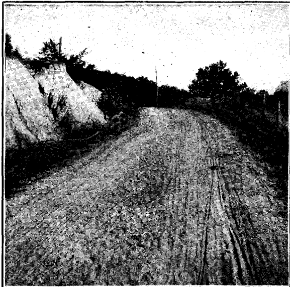
View on Bloomington-Columbus Pike, near Stobo P. O. Foundation, limestone; top-stream gravel.
