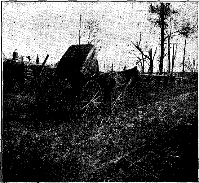
Showing the effect of summer showers on road in the residual clay of Harrodsburg limestone.
