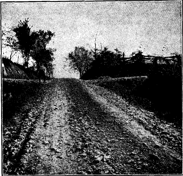
Stone road on which no screenings were used. One mile south Cross-Roads Church.
