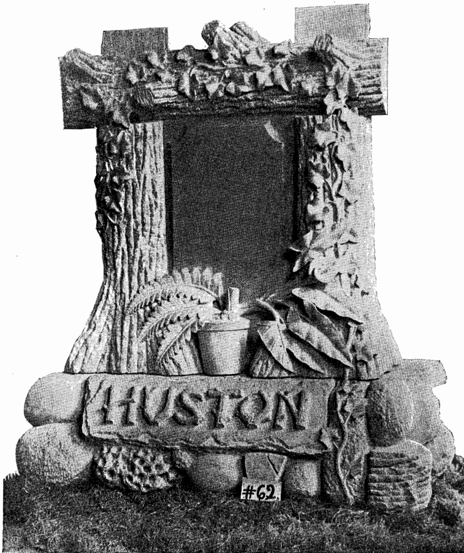
Fig. 12.—Carved from Bedford oölitic limestone, showing its adaptability to fine carving.
