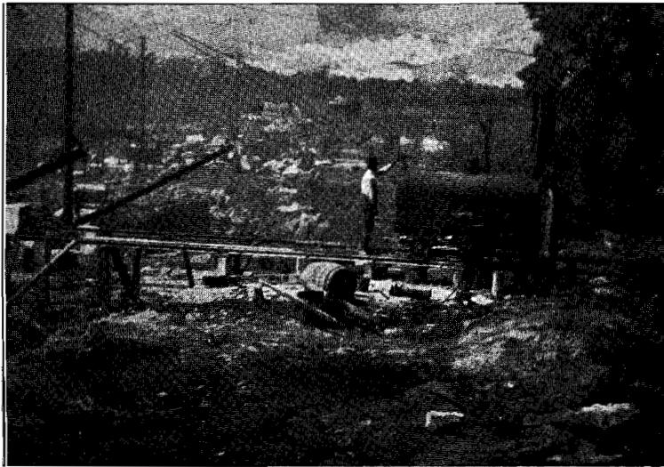
1. Hoosier quarry. Upper surface of the limestone after removal of the soil, showing also method of channeling on the side hill to get a level floor.
