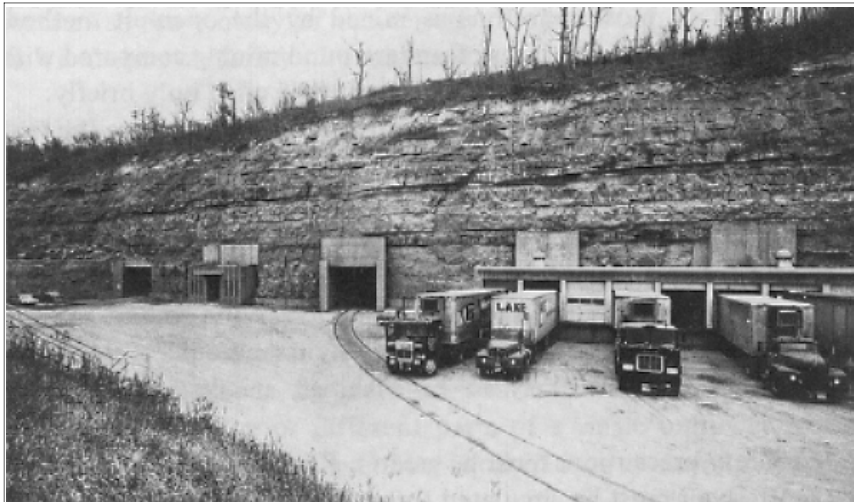
Figure 5. Inland Underground Facilities, Kansas City, Kans. The extensive mined-out areas of an active limestone tunnel mine (not shown here) are used for frozen-food storage, warehousing, manufacturing sites, office space, and vital records storage.
