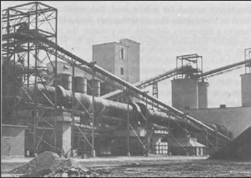
Figure. 13. Rotary kilns at the Marblehead Lime Co. plant near Gary, Ind.
