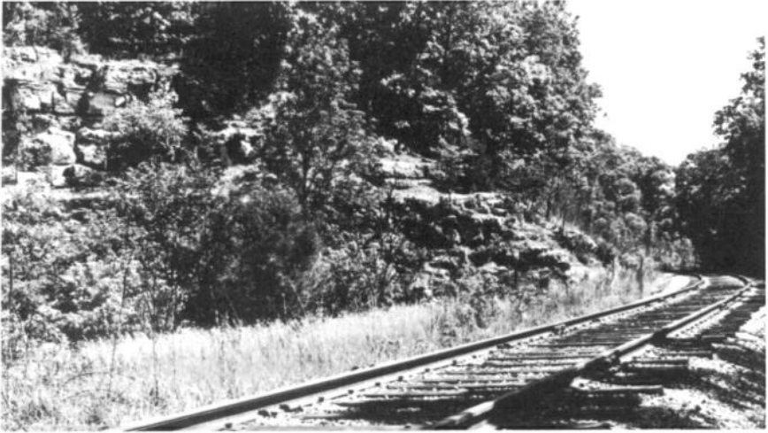
Figure 1. Abandoned railroad quarry exposing the Paoli and Ste. Genevieve Limestones in Orange County. This quarry is typical of many Indiana quarries that supplied ballast for building railroads about 1900. Although the life of these quarries was short, large quantities of stone were removed.
