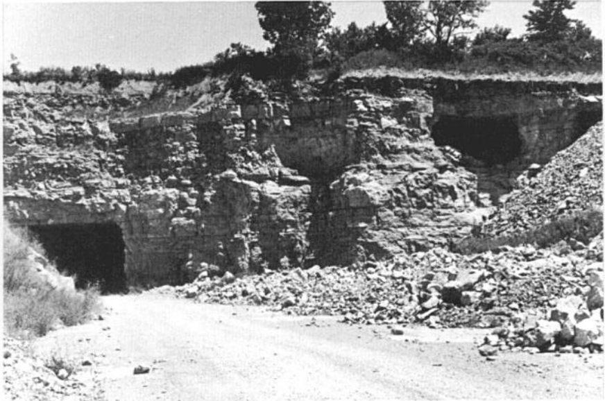
Figure 4. Inactive part of the Sellersburg Stone Co. quarry near Sellersburg, Clark County. Abandoned underground entries shown in the upper right of the photograph are in hydraulic limestones of the Speed Member of the North Vernon Limestone. Limestones of the Speed were used in many places in Clark, Floyd, and Jefferson Counties to manufacture natural cement until about 1900. Crushed stone was mined later from the mine shown in the lower left of the photograph after the upper mine had been abandoned and the quarry deepened.
