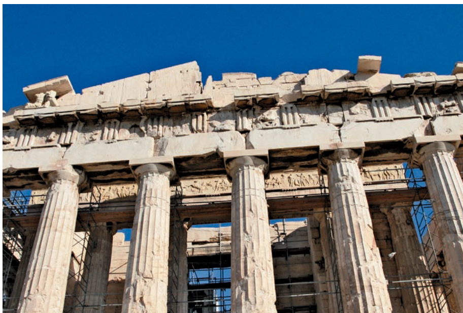
Fig. 16 : West façade of the Parthenon, Athens, with a view of the figures on the west frieze between the columns of the peristyle (Photo: author).
