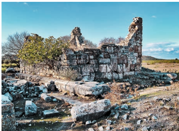
Fig. 7 : Heroon II. View from NE with marble foot profile of Roman podium front overbuilt by a medieval tower. Current state of preservation (photo author 10/2011).
