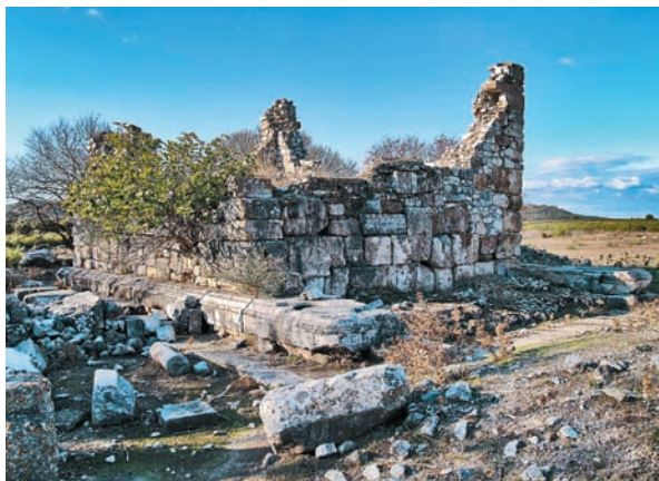
Fig. 7 : Heroon II. View from NE with marble foot profile of Roman podium front overbuilt by a medieval tower. Current state of preservation (photo author 10/2011).
