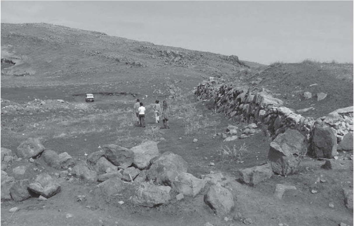
Fig. 14 : The inner battered face of the dam wall with the bank at right and a lower, inner, bank that the figures are traversing.
