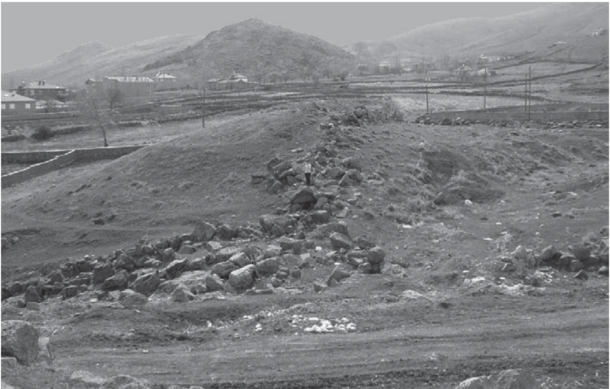
Fig. 15 : The dam from the east cut by the village road.
