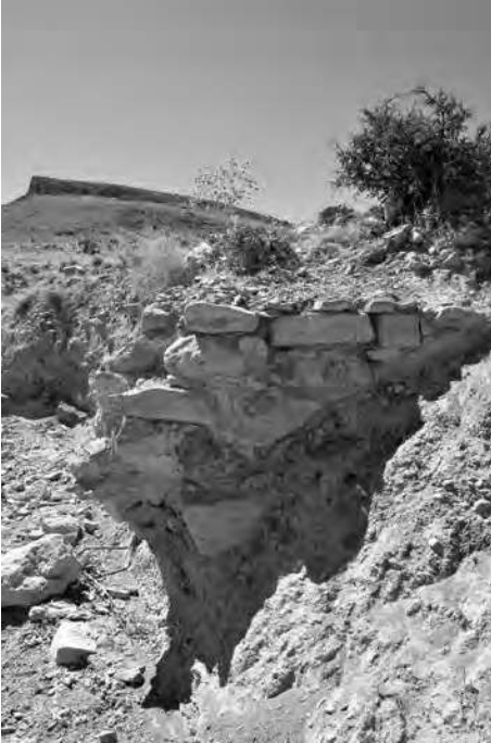
Fig. 32 : Walls (Late Antiquity) became visible after an erosion.
