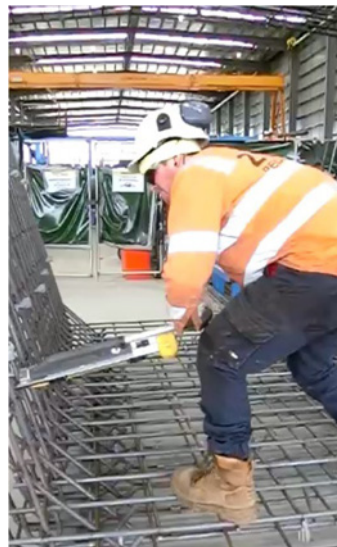
Figure 4 Use of the long handled stapler tool at ankle to knee level
