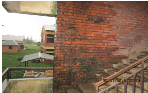
Figure1: Wall dampness during rainfall
