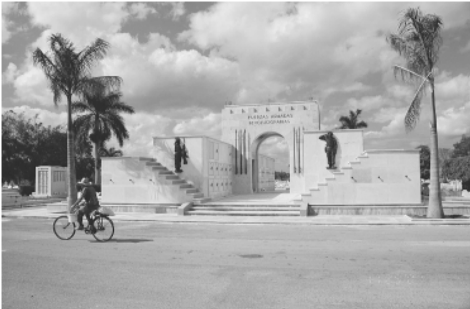
Away from the central avenues the cemetery begins to offer the historian something more than national heroes and a range of architectural styles from classical to modernist to Renaissance Mausoleum and monument to the Armed Revolutionary Forces, Cementerio Colón
