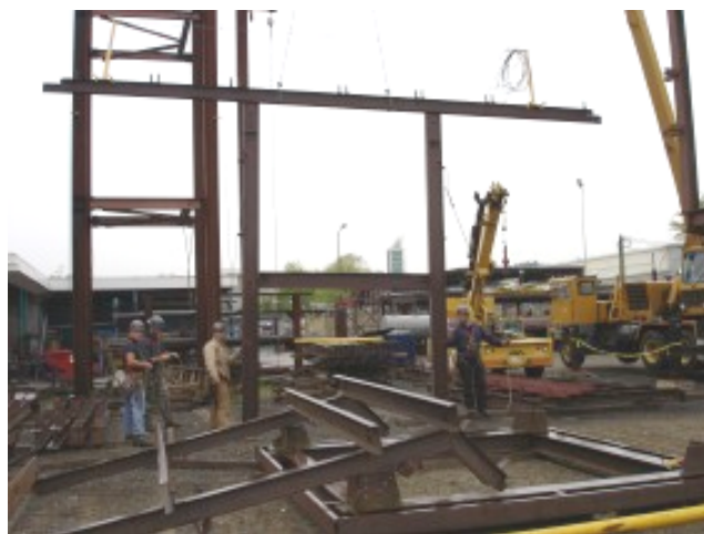
Figure 1: The four beams, assembled and being lifted by a two-choker sling
