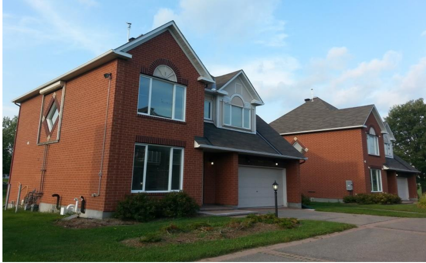
Figure 2.1: Canadian Centre for Housing Technology (CCHT) twin houses
