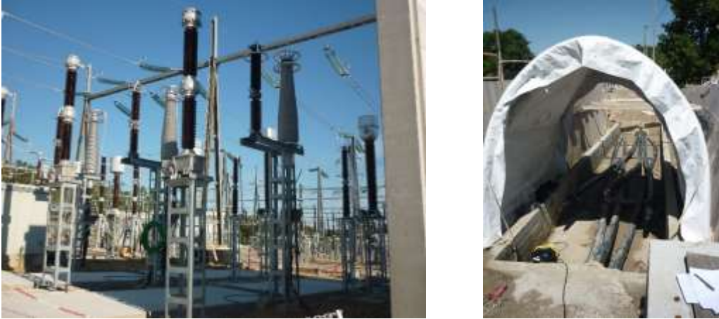
Figure 2.35 Sending and receiving end sites for surge field test of a major section of the RTE 225 kV cable.
