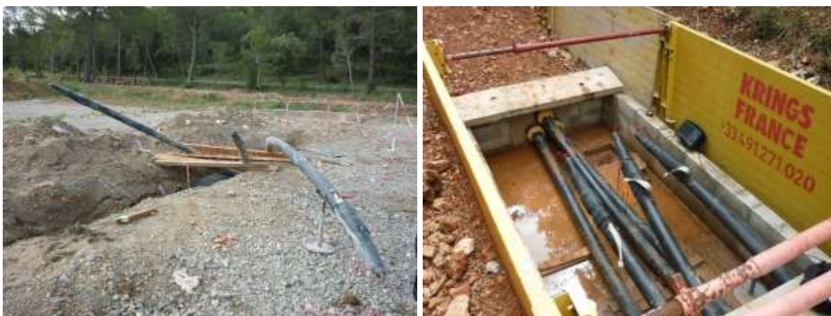
Figure 2.34 Sending and receiving end sites for surge field test of a minor section of the RTE 225 kV cable.
