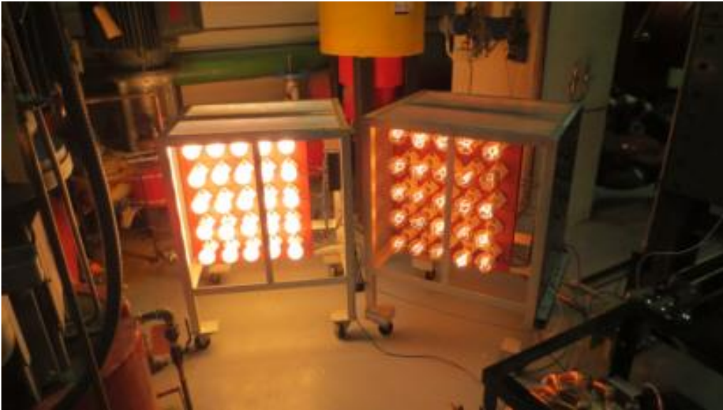
Figure 2.33 Carbon filament light bulb system to commission the electrical power.
