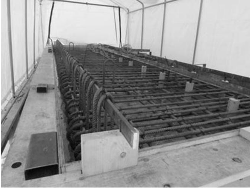
Figure 5-9: Slab Reinforcement and Anchor Support
