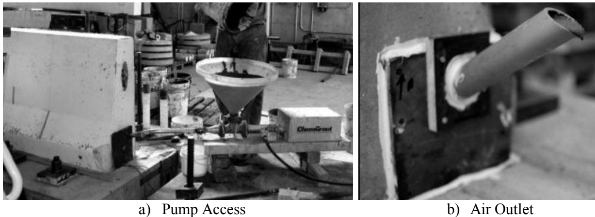
Figure 5-34: Mortar Injection, Pump Access and Air Outlet from Duchesneau (2010)
