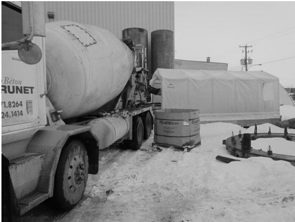
Figure 5-10: Truck Assess for Slab Casting
