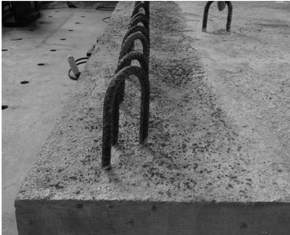
Figure 5-11: Exposed Aggregate Surface on Slabs
