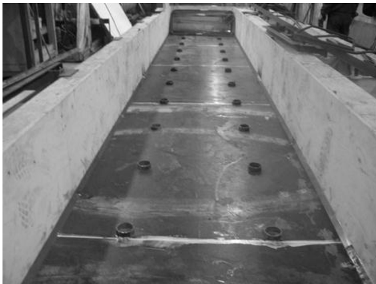
Figure 5-7: Block Formwork
