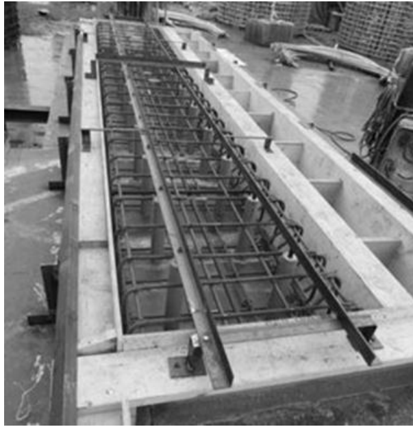
Figure 5-8: Block and Steel Bracing for Post-Tensioning Ducts
