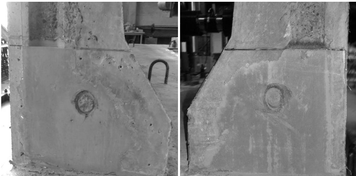
Figure 5-29: Ends of Hollow Recess after Injection
