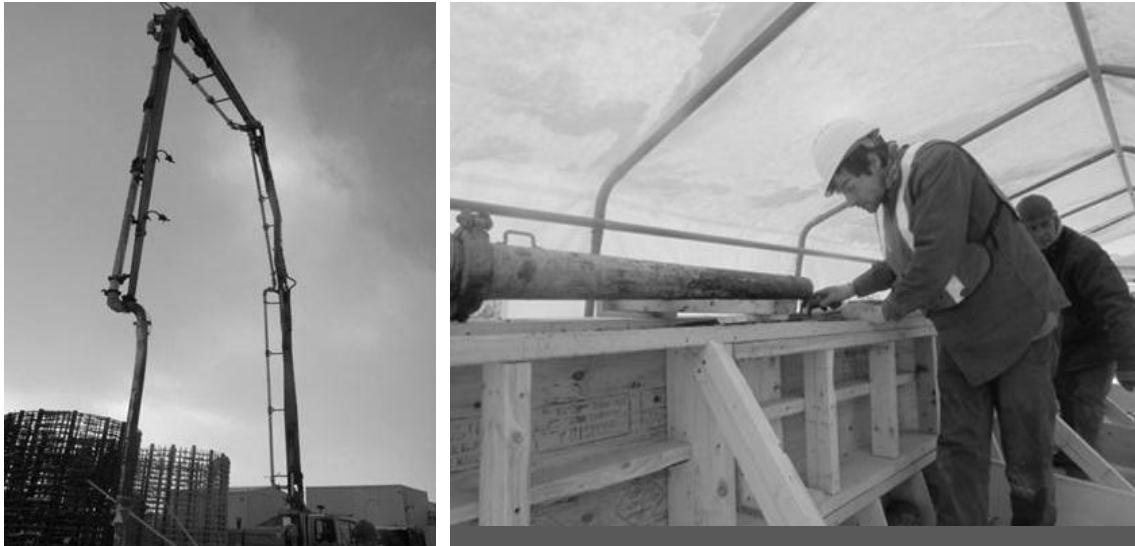
Figure 5-13: Barrier Pour with Industrial Pump
