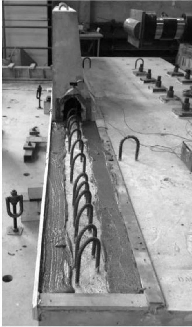
Figure 5-26: Mortar Bed for Precast Barriers
