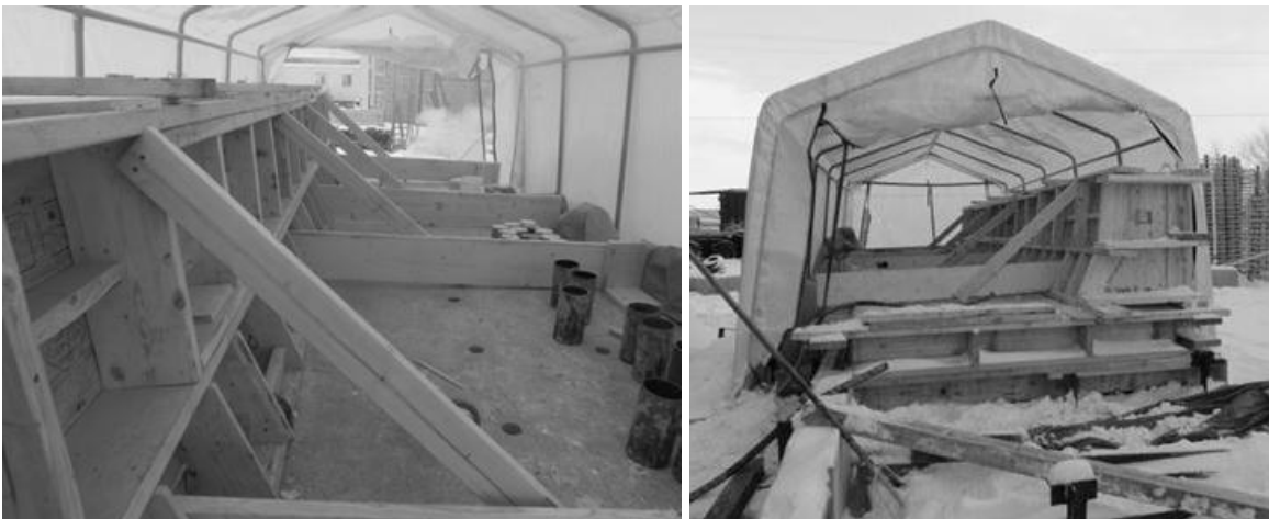
Figure 5-12: Formwork Assembly and Fixation, Cast-in-place Barrier
