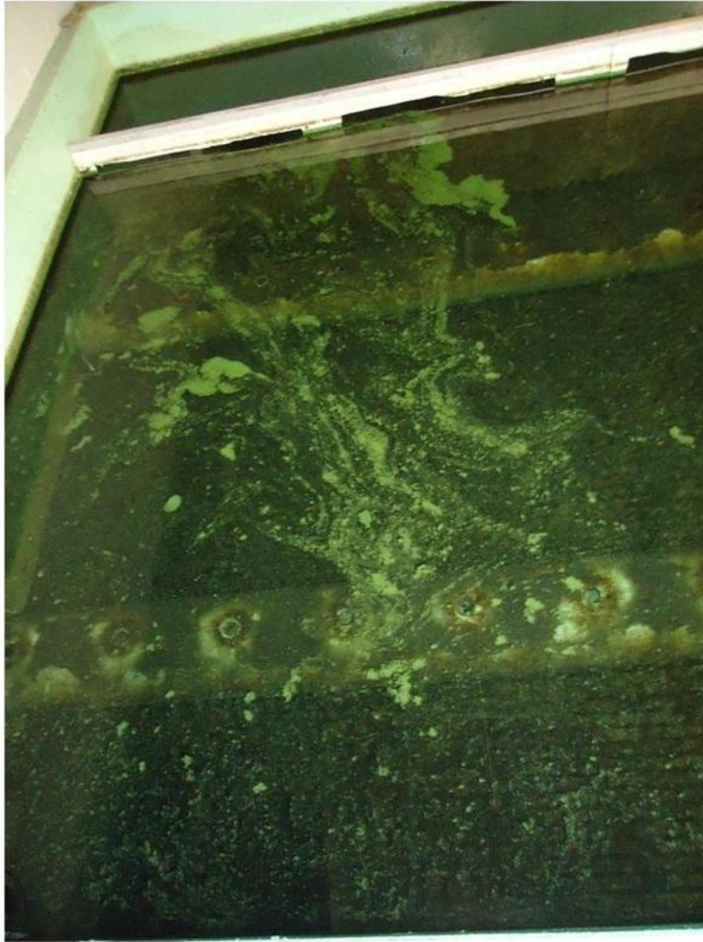
Figure 10.4: Accumulation of potentially toxic CB cells inside the studied DWTP in Quebec (Canada)
