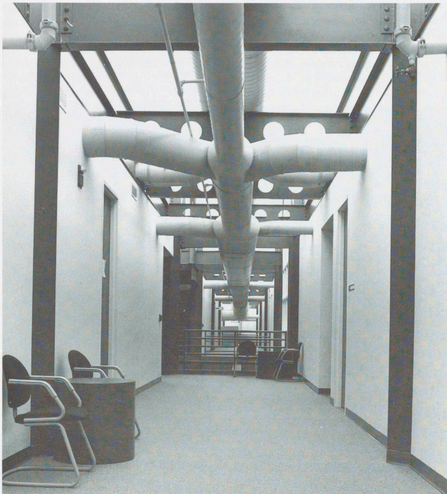
A second floor hallway of the incubator.
