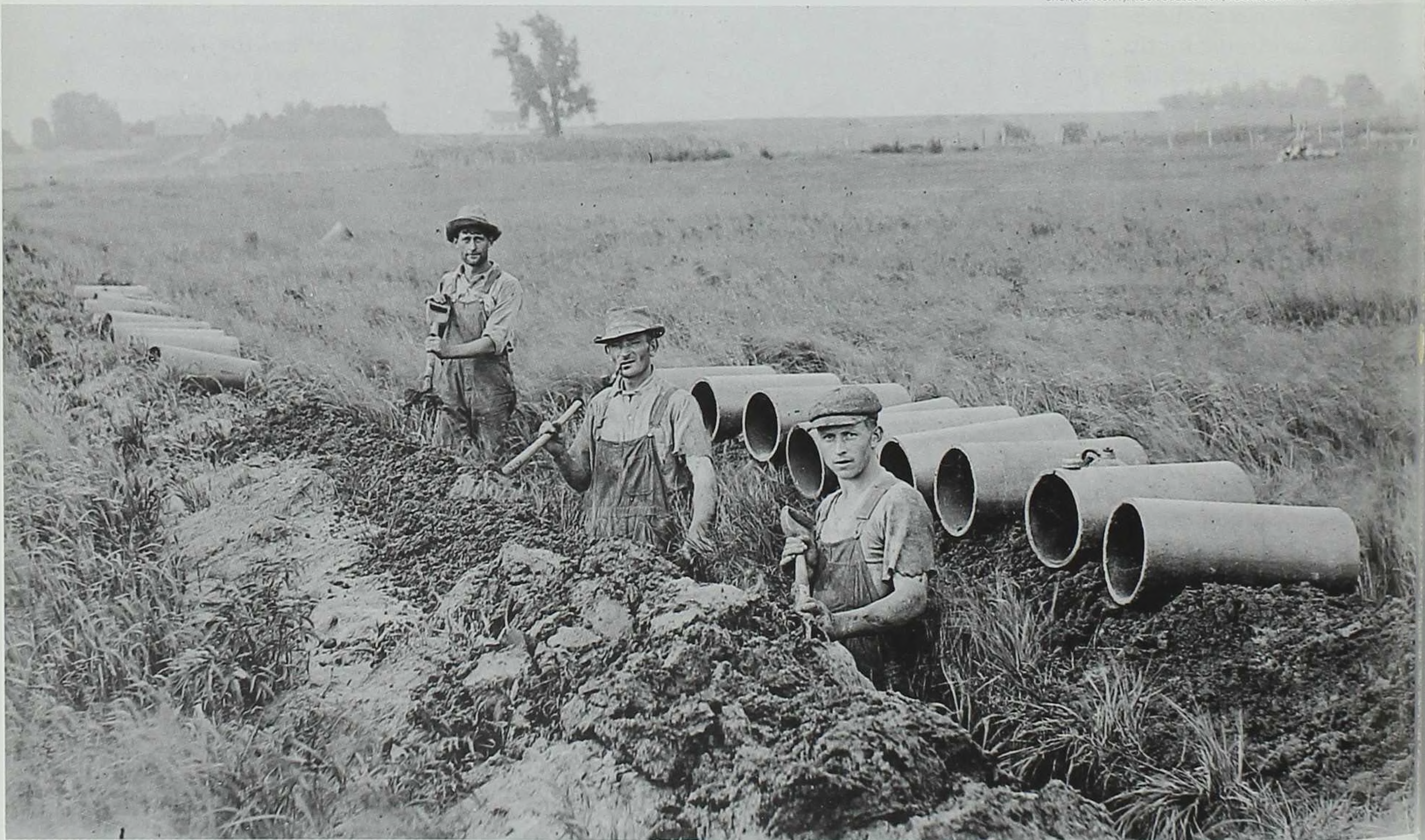
In north-central and northwestern Iowa, where the land was particularly flat, tile was laid to drain sloughs and other wetlands.
