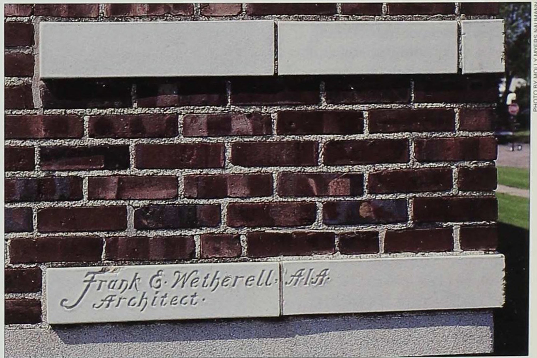
W etherell's signature on Lincoln School, in terra cotta.
