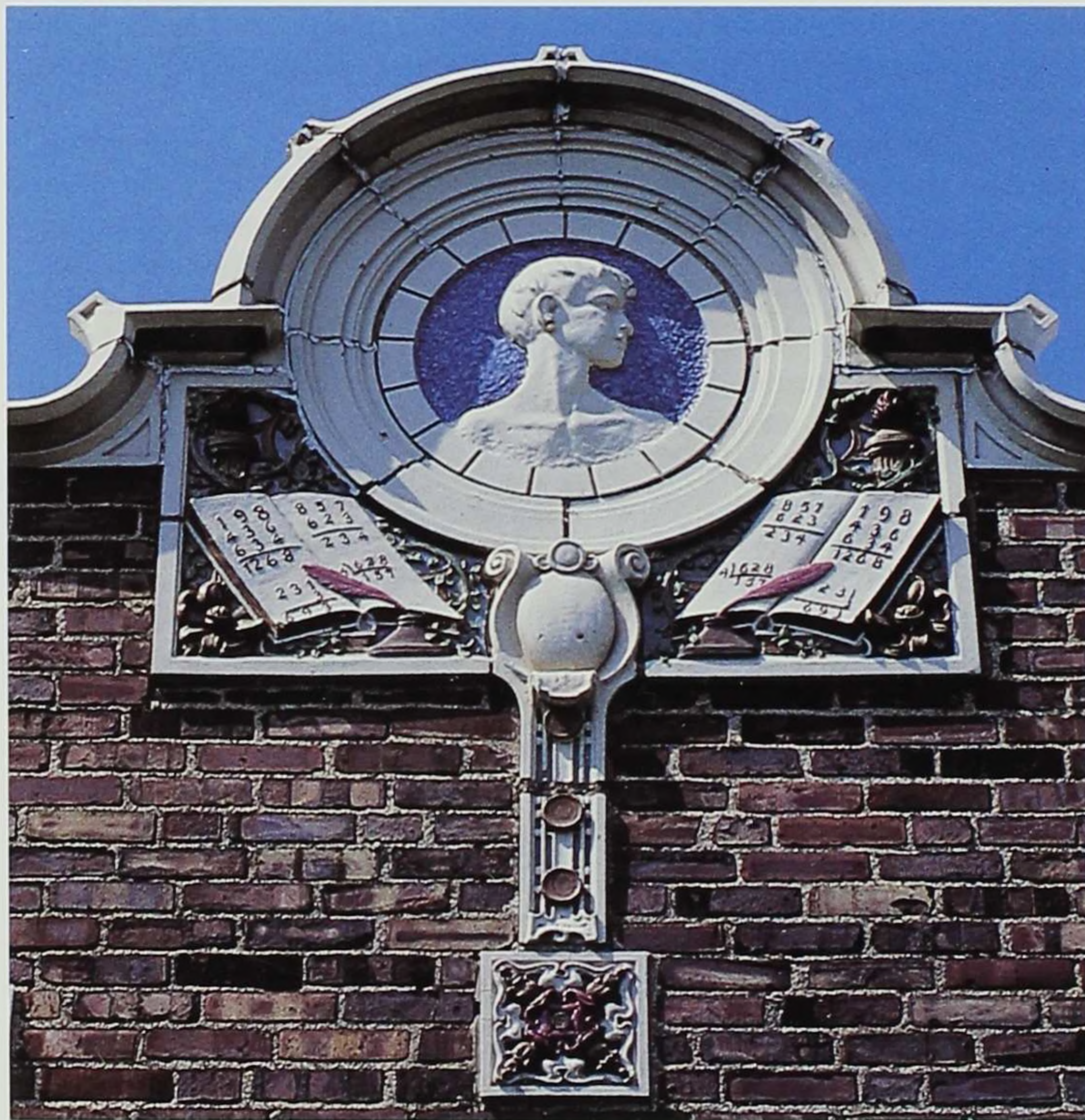
T erra cotta profiles of two students (above and right) punctuate the roof line of Lincoln School. Social thinkers believed that the architectural character of a modern school should express “the spirit of education,” as one educator put it, and create “an atmosphere of invitation to participate in the learning process.”
