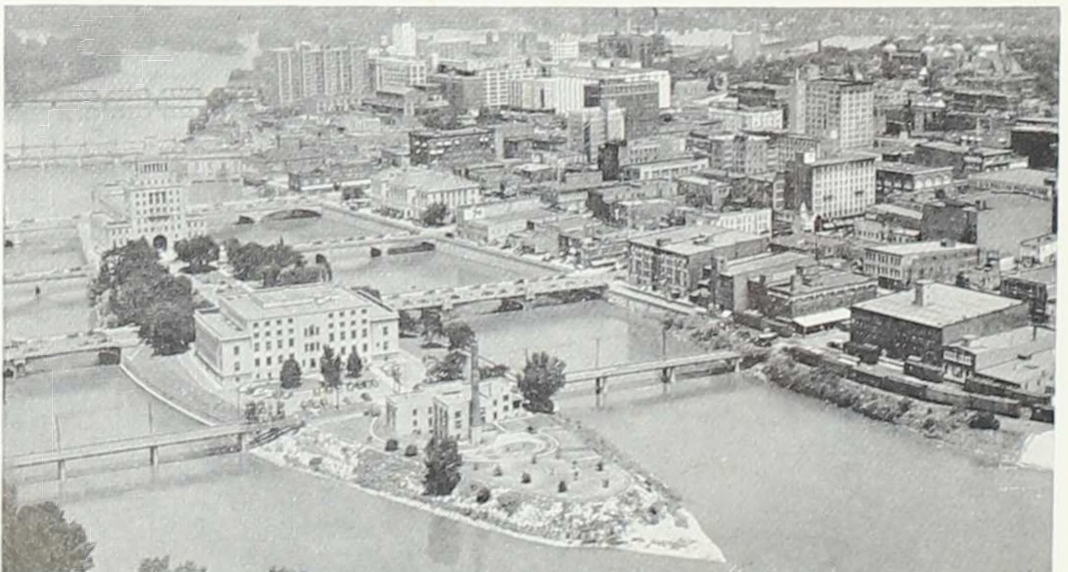
County and municipal buildings are located on an island at Cedar Rapids.
