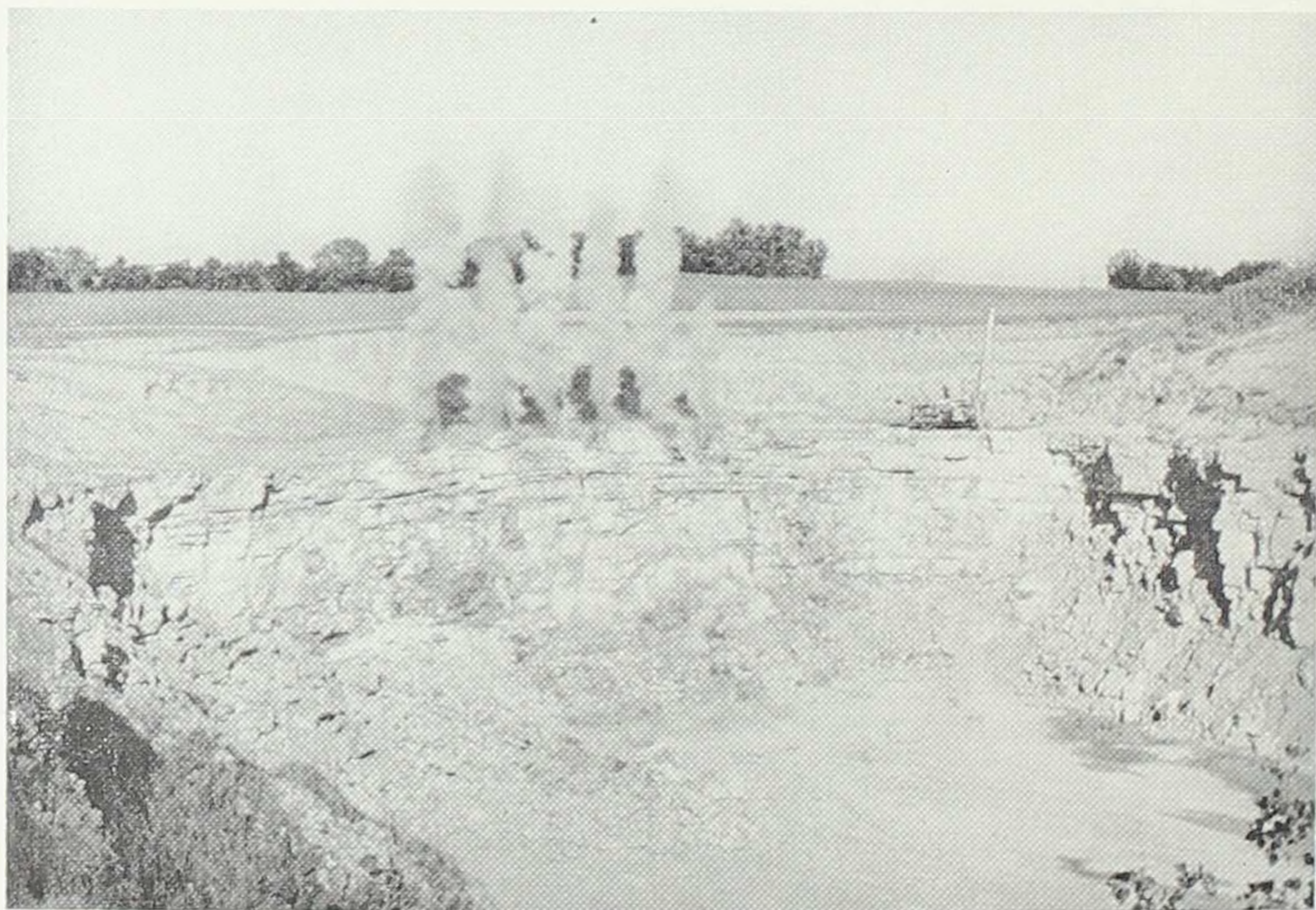
Explosives are set off in the rock; drilling machine at right of explosion.
