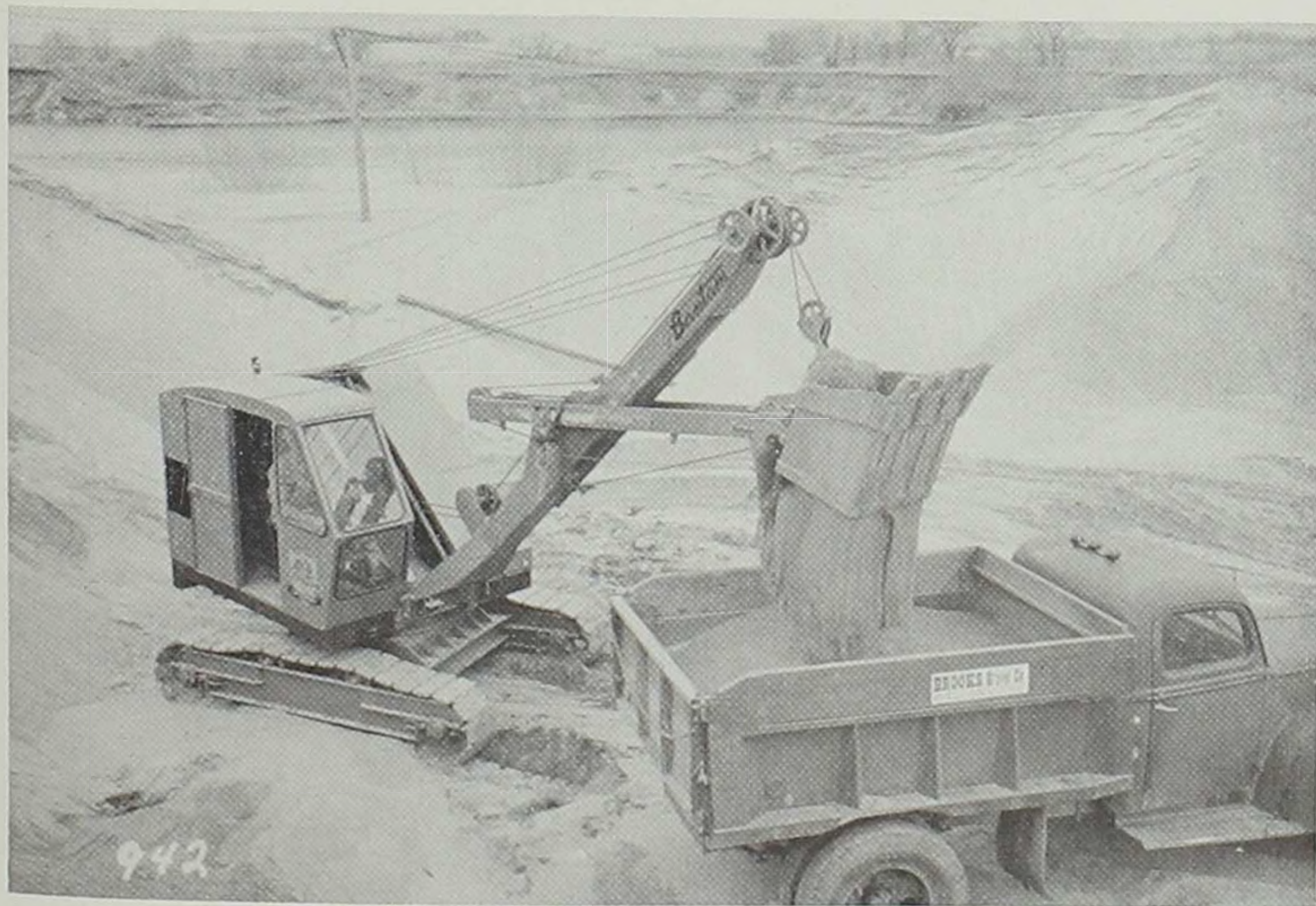
Shovel working in rock quarry loading stock-pile material.
