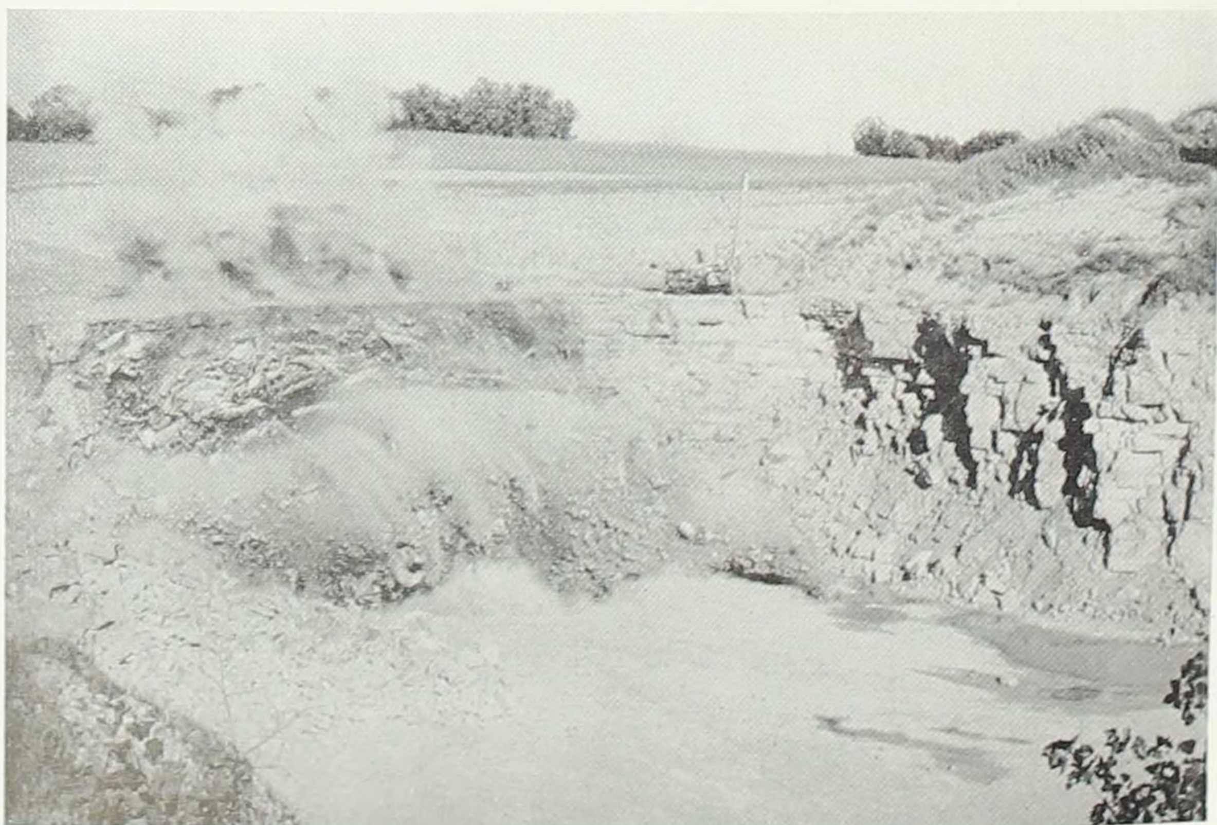
The results of the blast. Broken stone is used in highway construction and for other commercial purposes.
