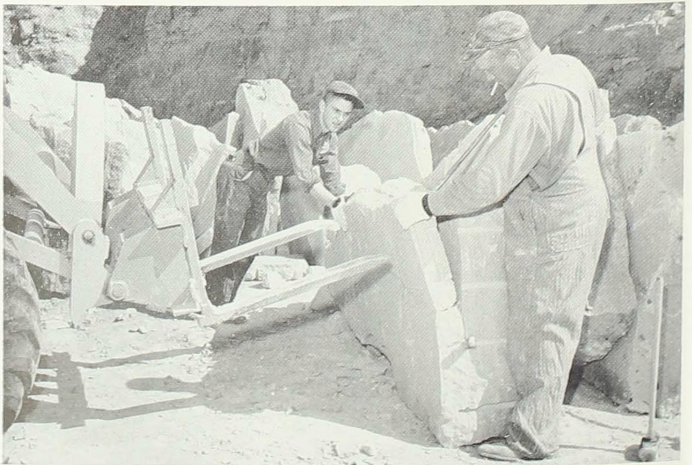
Slab of Anamosa limestone being lowered onto a fork lift.
