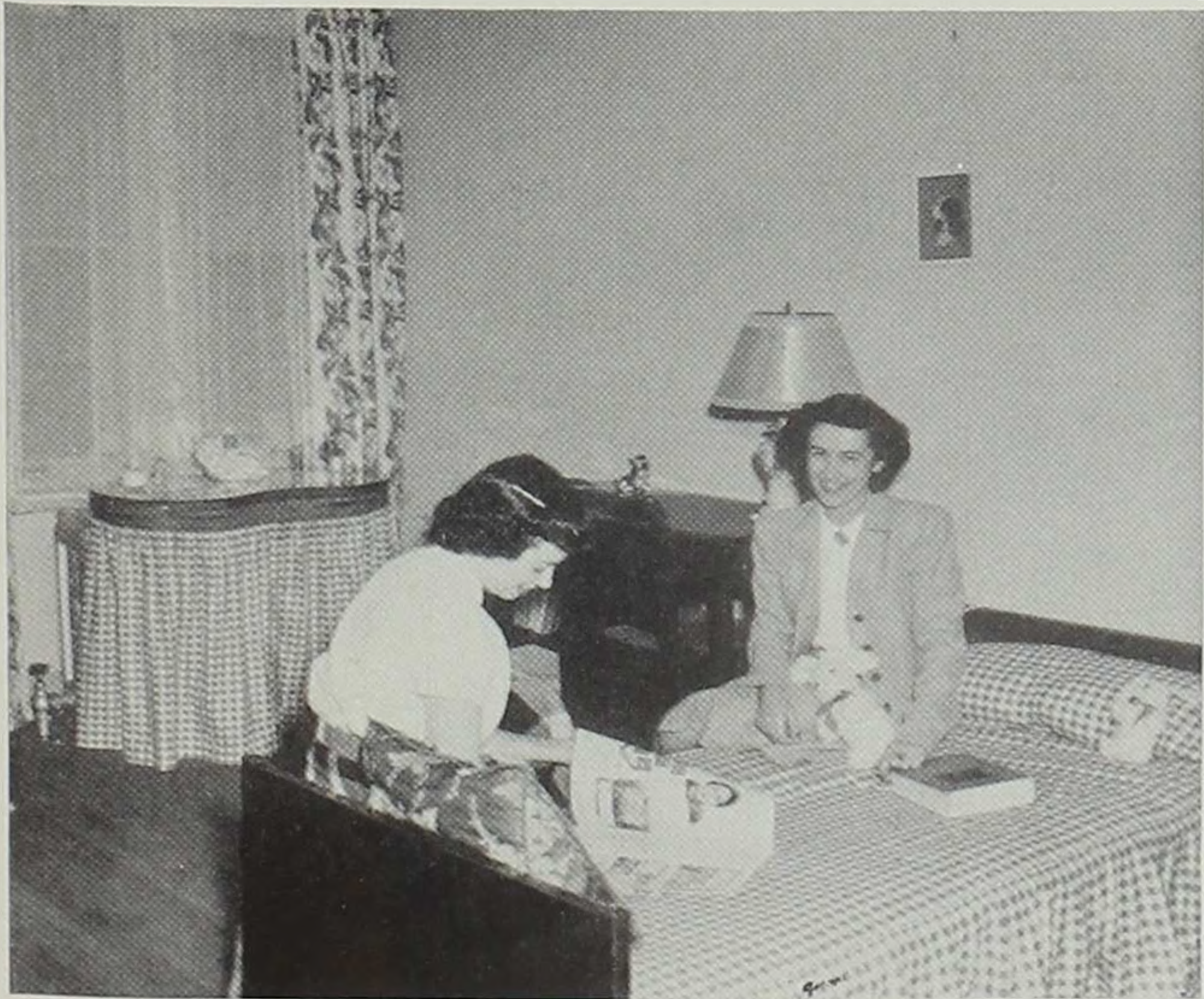
ROOM IN BALLARD HALL
