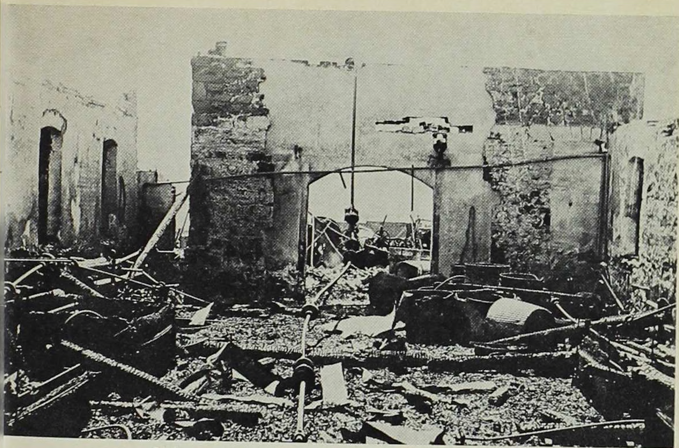
A disastrous fire destroyed a woolen mill at Amana.
