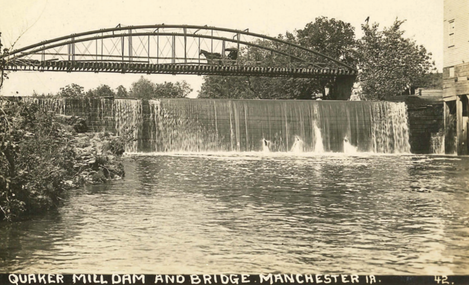
Quaker Mill dam and bridge, circa 1900–1910 (Robert Ungs).
