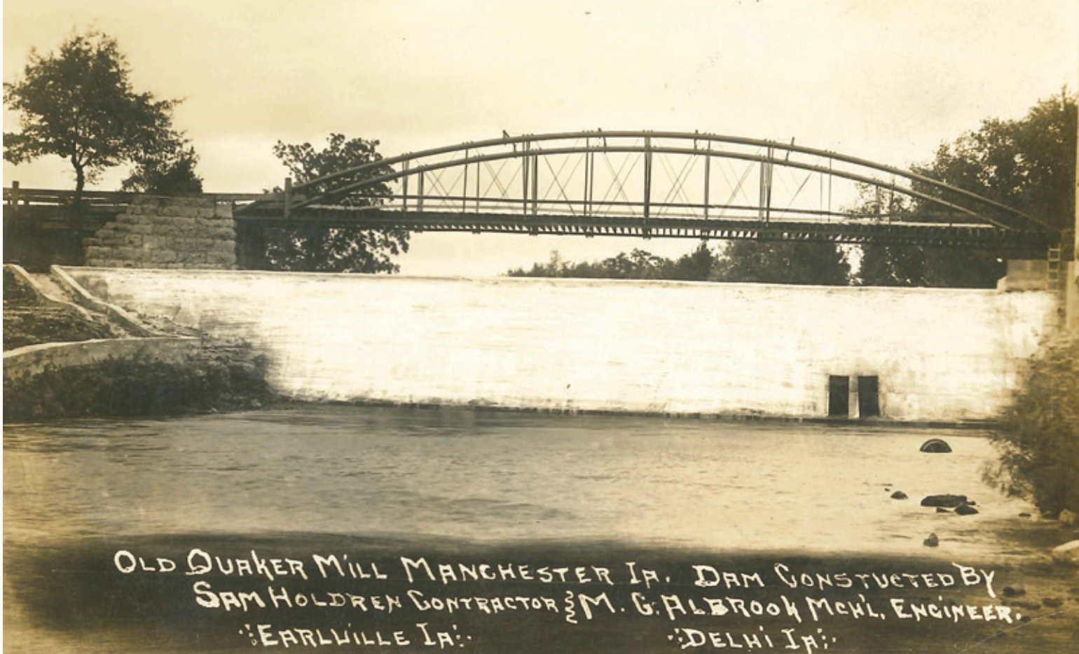
Quaker Mill Dam and bridge, circa 1914–1922, showing 1914 concrete dam (Robert Ungs).
