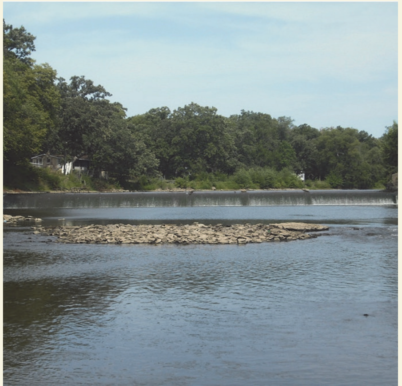
View of Littleton Dam from downstream, 2012 (OSA).
