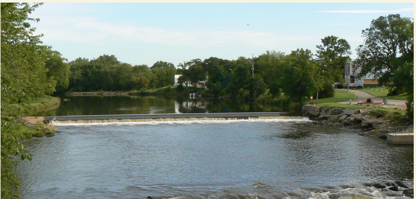
View of Quasqueton Dam from downstream, 2009 (from USFWS).
