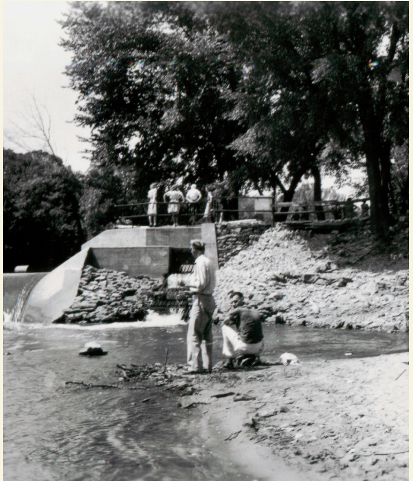
View of 1938 fishway at Littleton Dam, 1939 (from LCHS-FFPC).
