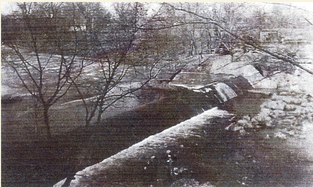
View of Littleton Dam, 1934 (from LCHS).
