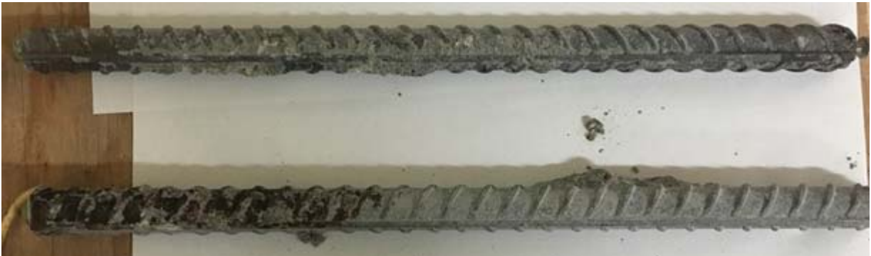
Figure 49 — Cracked beam MMFX(4%)-5 bottom bars after 96 weeks
