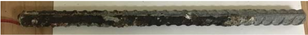
Figure 48 — Cracked beam MMFX(4%)-5 top bar after 96 weeks
