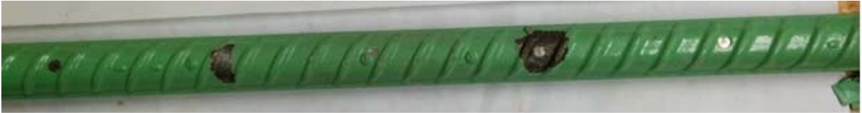
Figure 32 — Southern Exposure MMFX-ECR(2%)-5 bottom bar after disbondment test after 96 weeks
