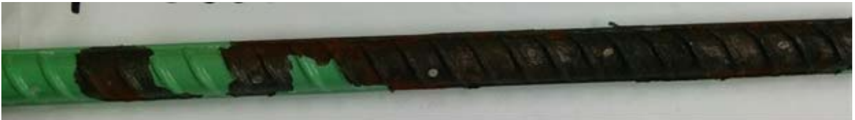
Figure 51 — Cracked beam MMFX-ECR(2%)-2 top bar after disbondment test after 96 weeks
