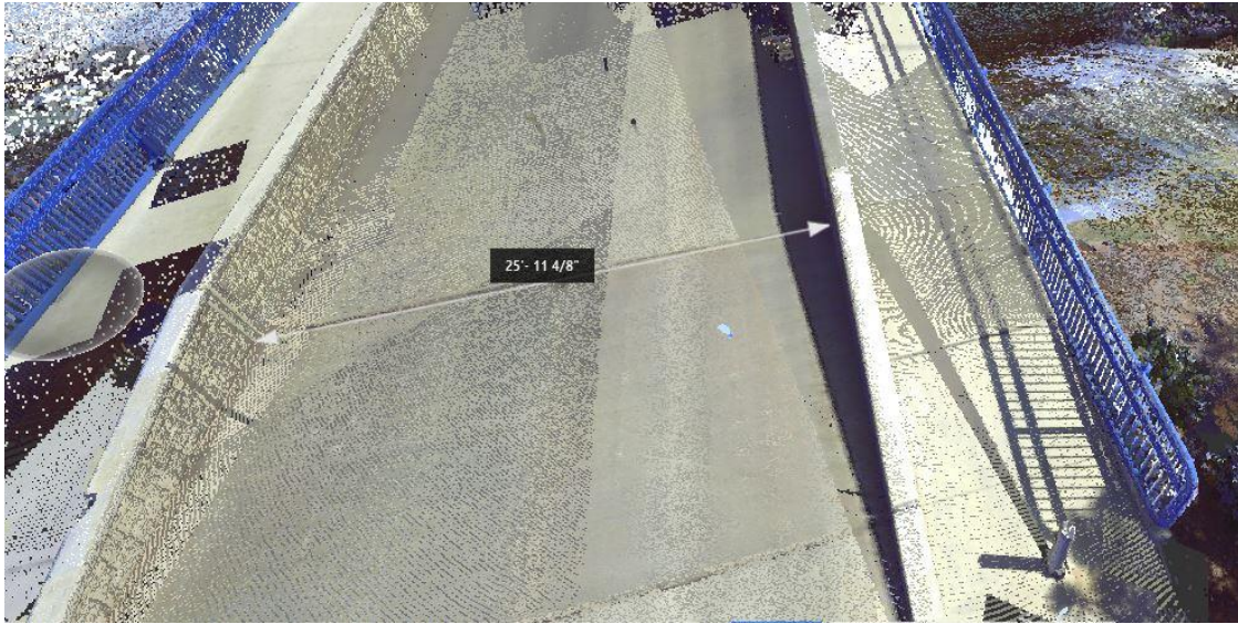
Figure 5.14a: Bridge roadway width from scan data
