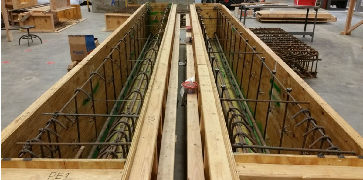
Figure 1.8: Reinforcement cages with conventional stirrups (left) and headed bars (right) as shear reinforcement
