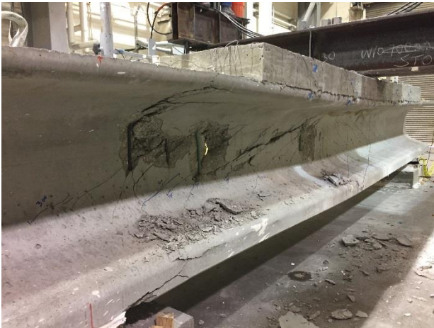
(c) Specimen after Failure
