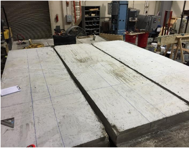
(a) Chalk Lines Indicating the Location of Saw-Cuts
