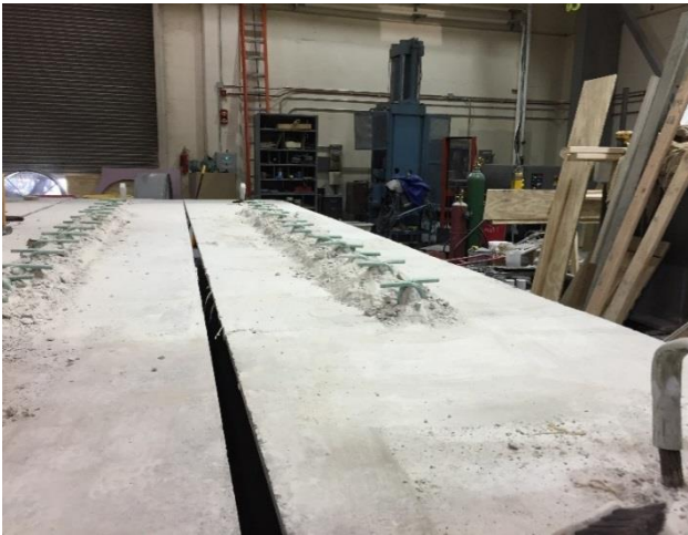
(c) Prior to use of Variable Impact Demolition Hammer
