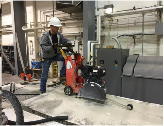
(b) Longitudinal Saw-Cuts
