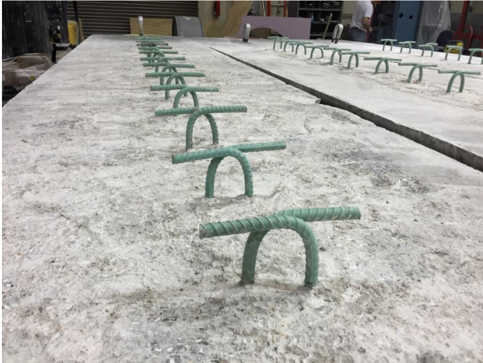
Figure 4.12: Girder #3 Surface after Deck Removal (Originally Fully Roughened)
