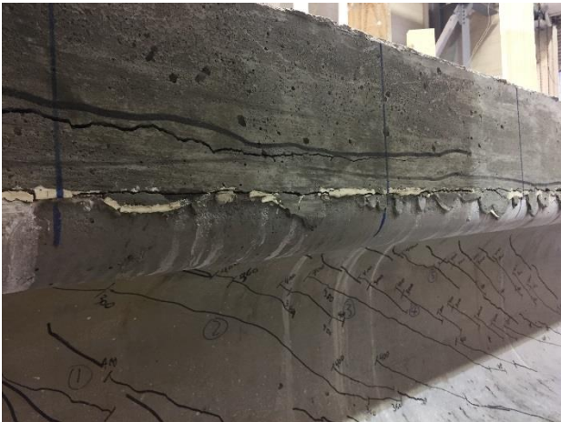
(c) Horizontal Crack Through Deck After Failure (West Side)
