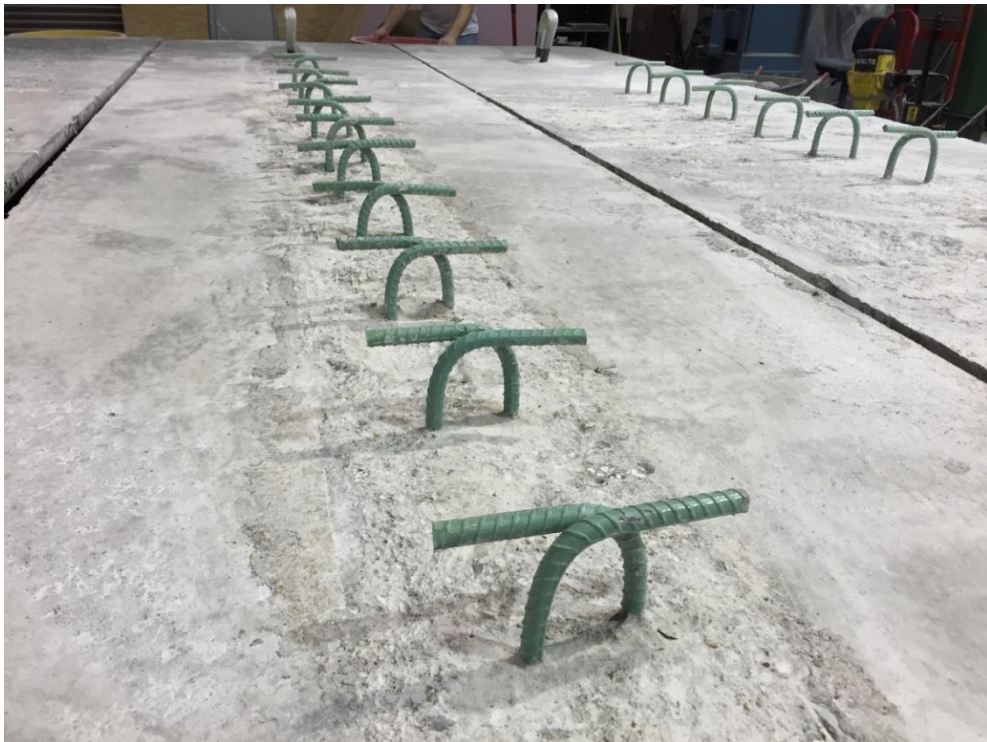
Figure 4.13: Girder #2 Surface after Deck Removal (Originally Partially Roughened with Roofing Felt over the Flange Tips)
