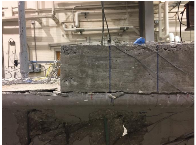
(f) Permanent Slip between Girder and Deck after Failure
