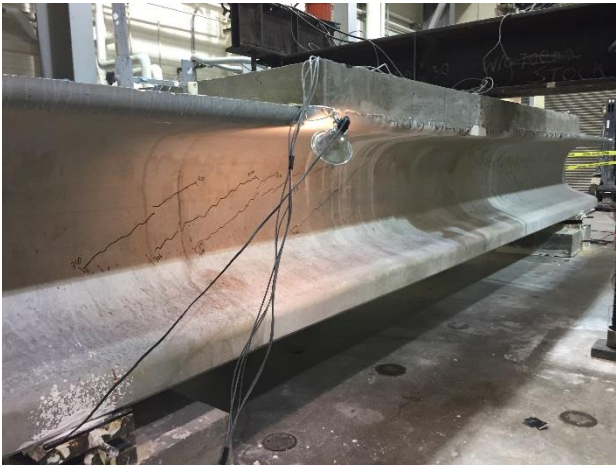
(a) Cracking at 300 kips
