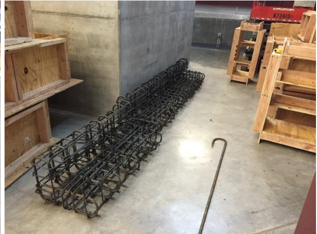
(b) Reinforcement Cages
