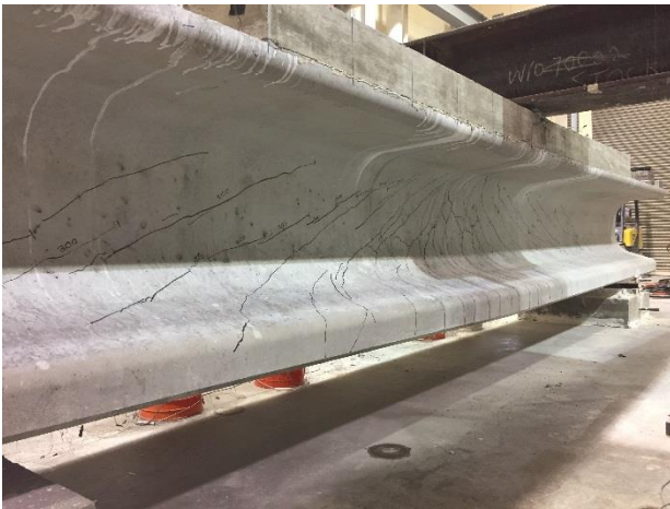
(a) Cracking at 400 kips
