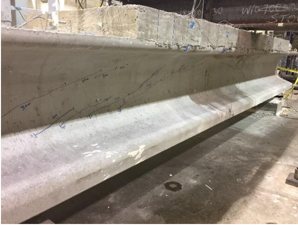
(a) Web Shear Cracks at 205 kip
