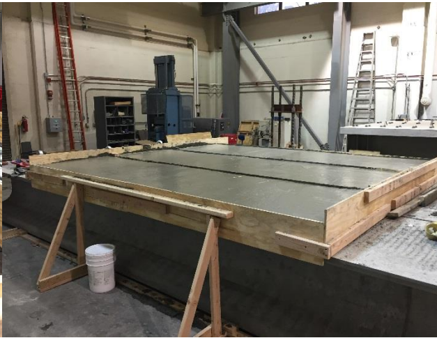
(b) Concrete Deck after Finishing
