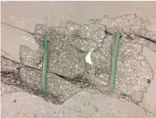
(e) Girder Web after Failure
