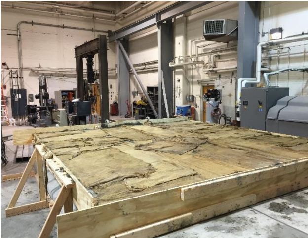
(c) Concrete Deck Curing
