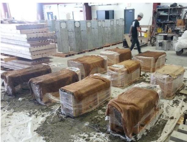
(e) Concrete Curing
