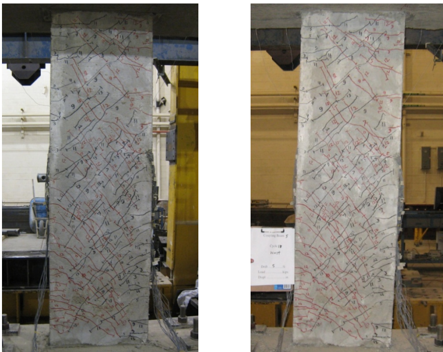
Figure 7: Damage in coupling beam with aspect ratio of 3.3 at 3% (left) and 5% (right) drift.
