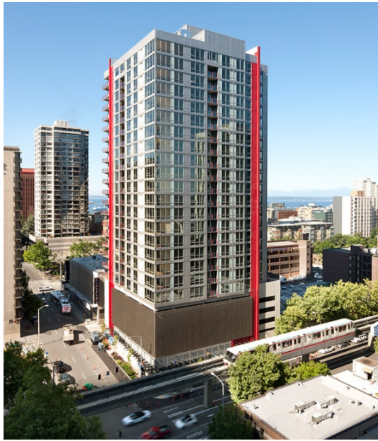
Figure 8: The Martin , a core-wall structure with HPFRC coupling beams in Seattle, WA, USA.
