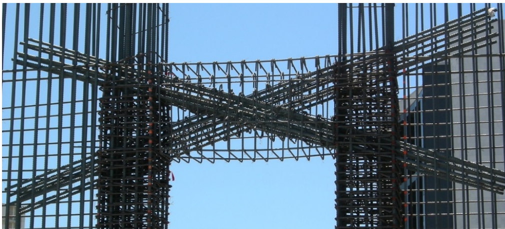
Figure 1: Typical design of earthquake-resistant coupling beams.
