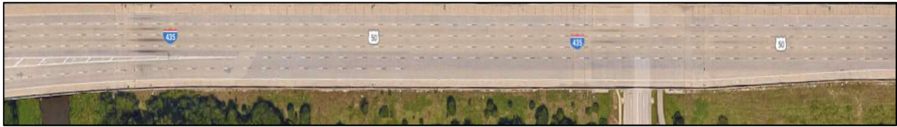
Figure 18: I-435 East Bound at Roe Avenue (Google Maps)
