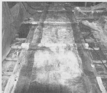
Fig. 5—Cast and curing operations.
