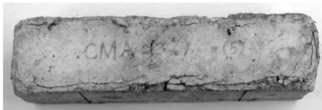
Fig. 7—Specimen subjected to 95 weeks of exposure to 1.06 molal ion concentration solution of CMA.
