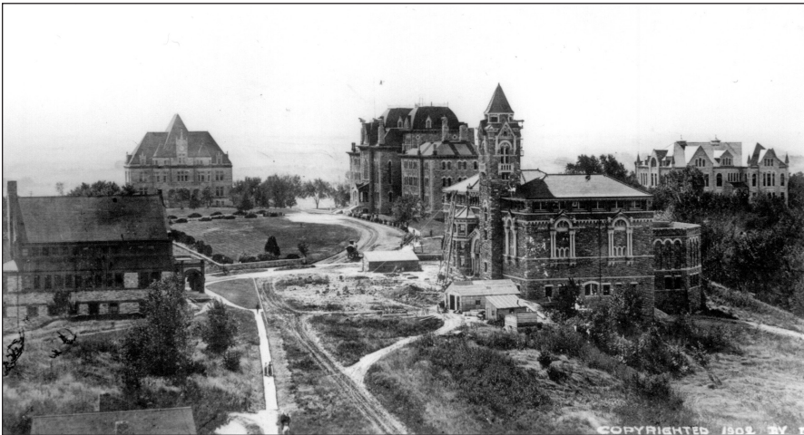
When Kate attended the University of Kansas in the early years of the twentieth century, KU was in a significant expansion phase. In this photograph Dyche Hall is under construction, and old Fraser and Blake halls are to the south of Dyche.
