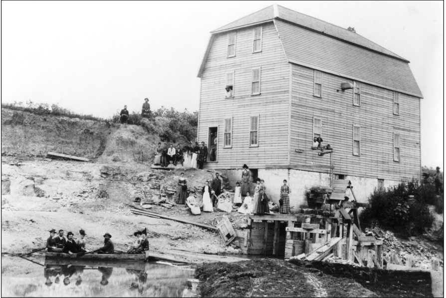
This flour mill was one of several saw- and flour mills in the Logan area owned by the Hansen family. Peter Hansen had the vision to know that lumber, other building materials, and flour would be needed by post-Civil War settlers.
