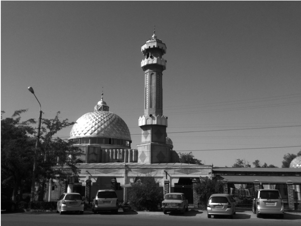
Figure 13: Bishkek Central Mosque (photo by author).
