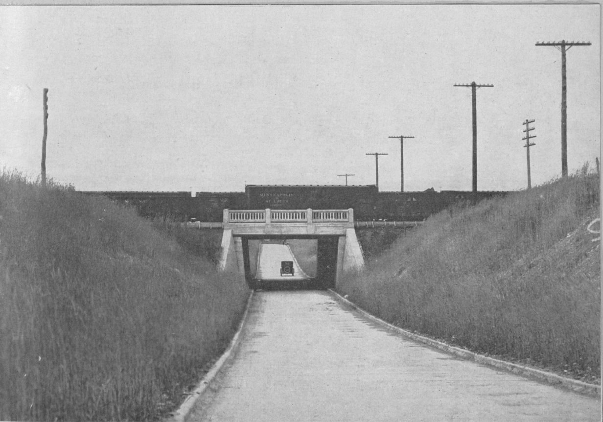
Figure 5 - Subway on Illinois Highway
