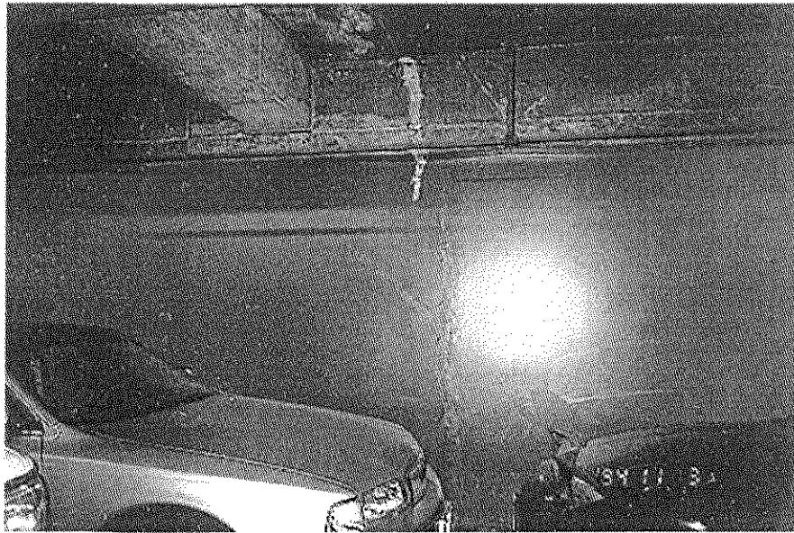
Figure 2-12. Wall after painted and repaired with epoxy (Naeim, 2000)
