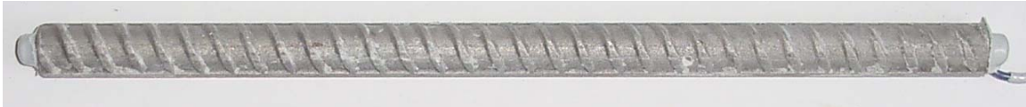
Figure 3.133 – 2205p bar used on top mat of cracked beam specimen, showing no corrosion products, at week 96.
