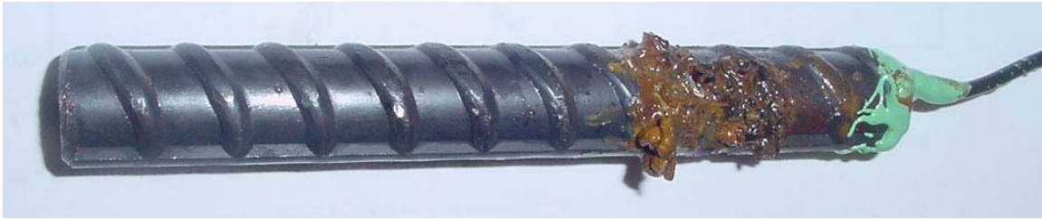
Figure 3.61 – Bare MMFX steel anode bar from group MMFX(1) showing corrosion products that formed above the surface of the solution at week 15.
