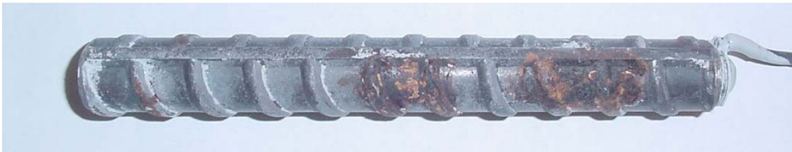
Figure 3.71 – Corrosion products on MMFX steel anode after removal of mortar cover at week 15.
