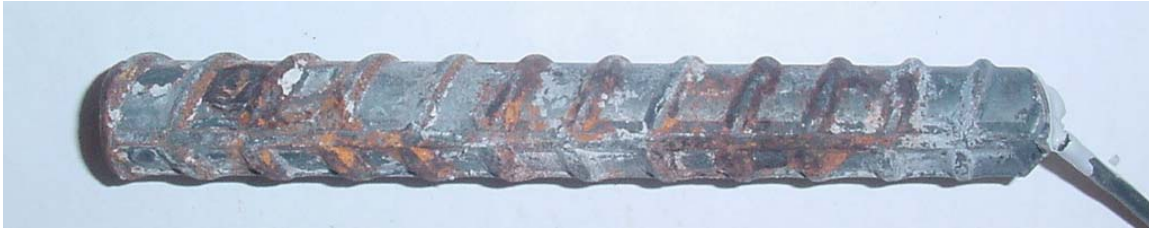
Figure 3.70 – Corrosion products on conventional steel anode after removal of mortar cover at week 15.
