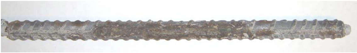
Figure 3.127 – Corrosion products on 2101(1) steel bar from top mat of cracked beam specimens at week 96.
