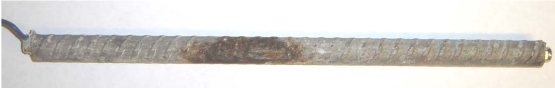
Figure 3.128 – Corrosion products on 2101(1)p steel bar from top mat of cracked beam specimens at week 96.
