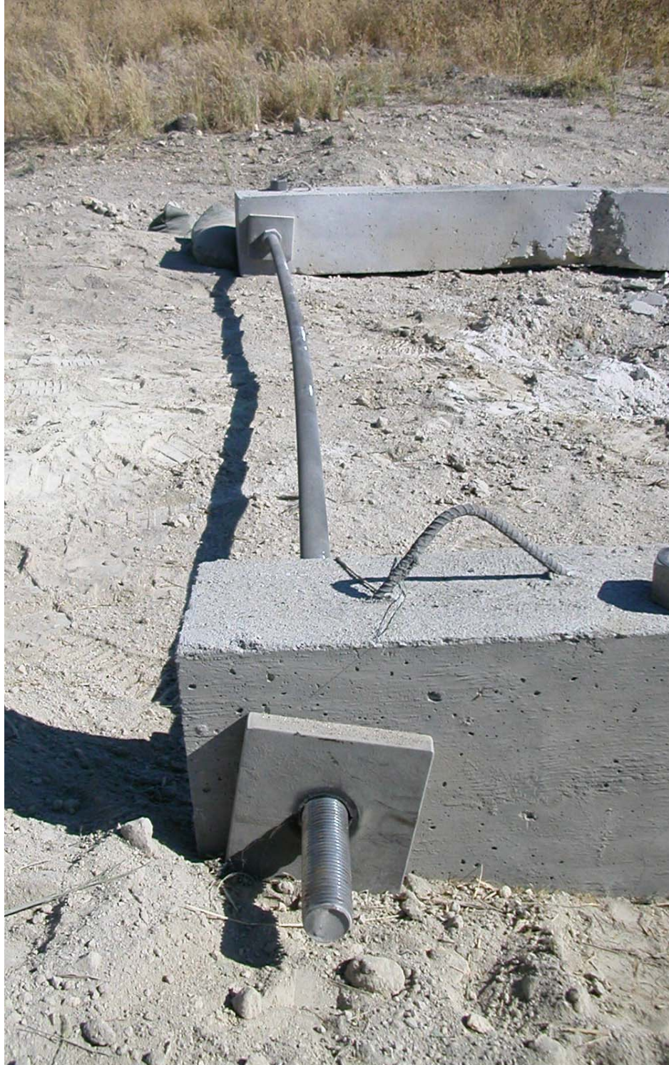
Figure A.15 –Set 3 following detonation of 15 lbs (6.80 kg) of C-4. Note the inward bow in the steel rod, following the blast, due to yielding of the concrete beams. A similar bow in the steel rod was observed on Sets 1 and 2 following their blasts.
