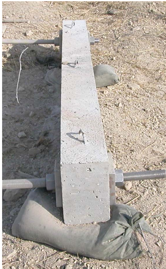
Figure A.22 – Beam 4B following detonation of 6.25 lbs (2.83 kg) of C-4. Note that the beam appears straight with no outward sign of yielding of the reinforcement within the beam.
