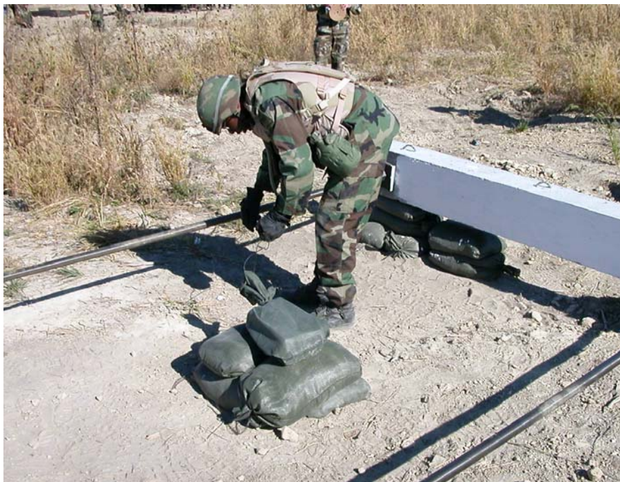
Figure A.12 – The C-4 charge was placed in an empty sandbag to protect it during transport from charge assembly area to the blast site. The charge was centered between the two beams and placed on sandbags to make it approximately level with the centerline of the two beams.
