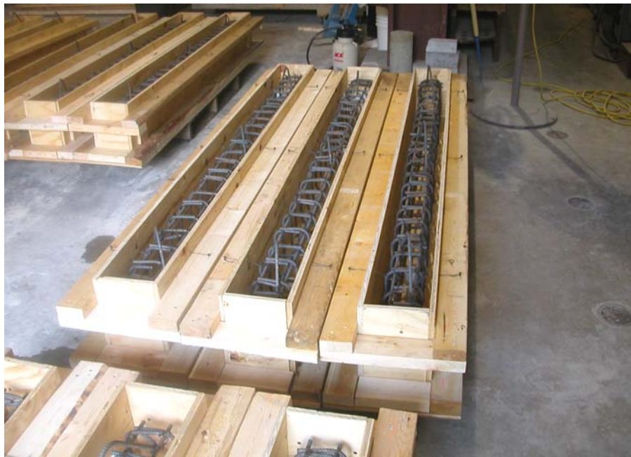
Figure A.4 – Forms prior to placement of concrete.
