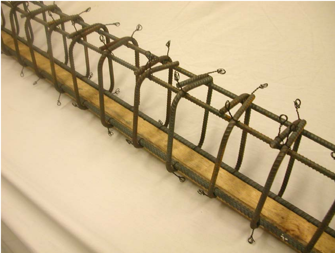
Figure A.2 – Reinforcing cage with horizontal reinforcement wire tied to stirrups, prior to the removal of the wood spacing jig.
