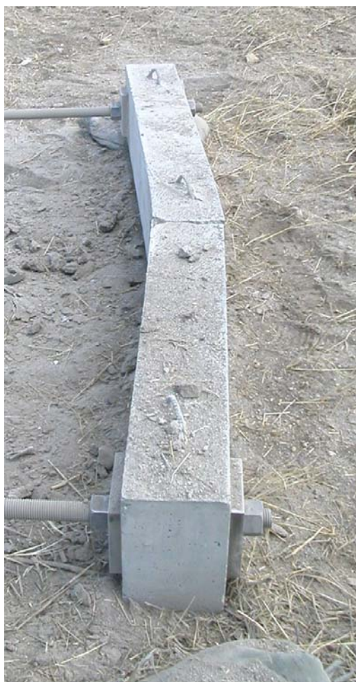
Figure A.20 – Beam 1B following detonation of 10 lbs (4.54 kg) of C-4. Note the outward bend due to the yielding of the concrete beams.
