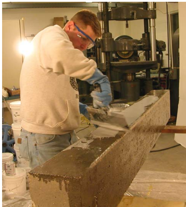
Figure A.42 – The MBRace Putty has a high viscosity and is applied using a steel trowel.
