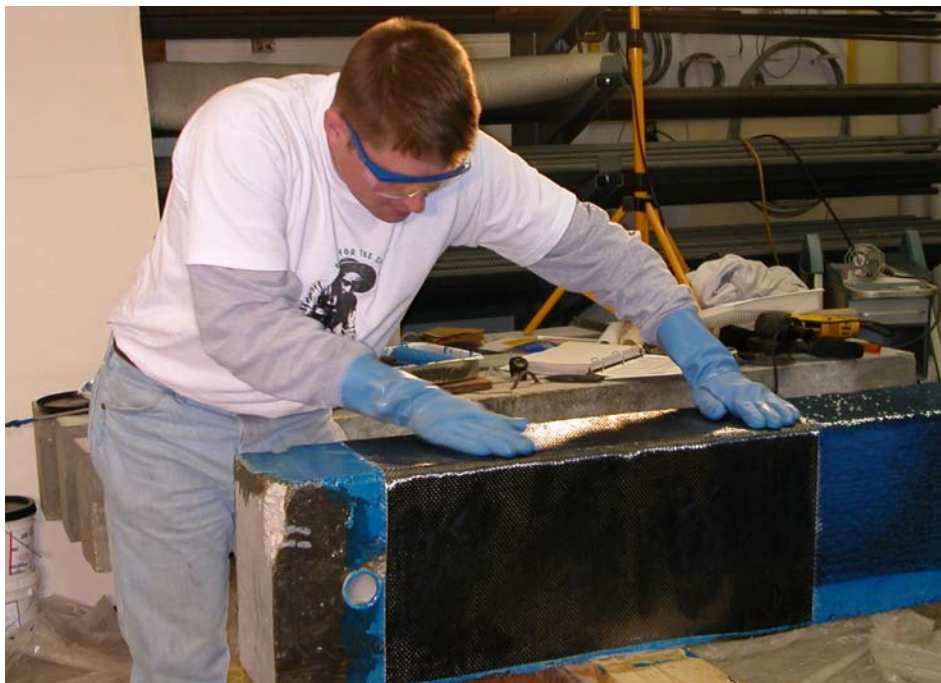
Figure A.50 – The fabric was smoothed to remove all air voids beneath it and the previous layers. Care was also taken to ensure the fibers in the fabric remained straight and properly oriented.
