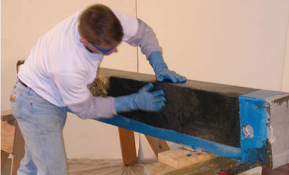
Figure A.47 –The first layer of carbon fiber fabric was applied running parallel to the beam’s primary axis. This layer of fabric provided tensile reinforcement to the beams.
