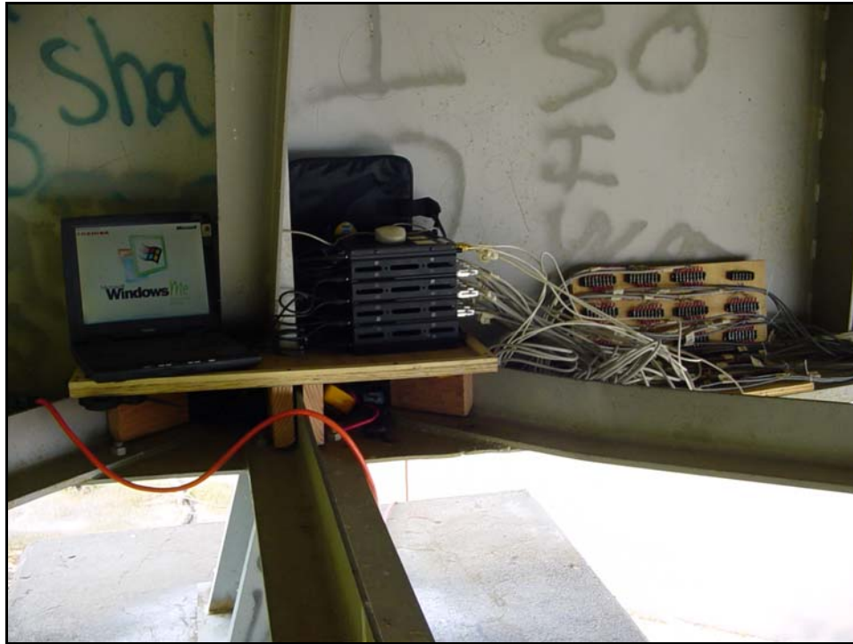
Figure C-5 Data Collection Station
