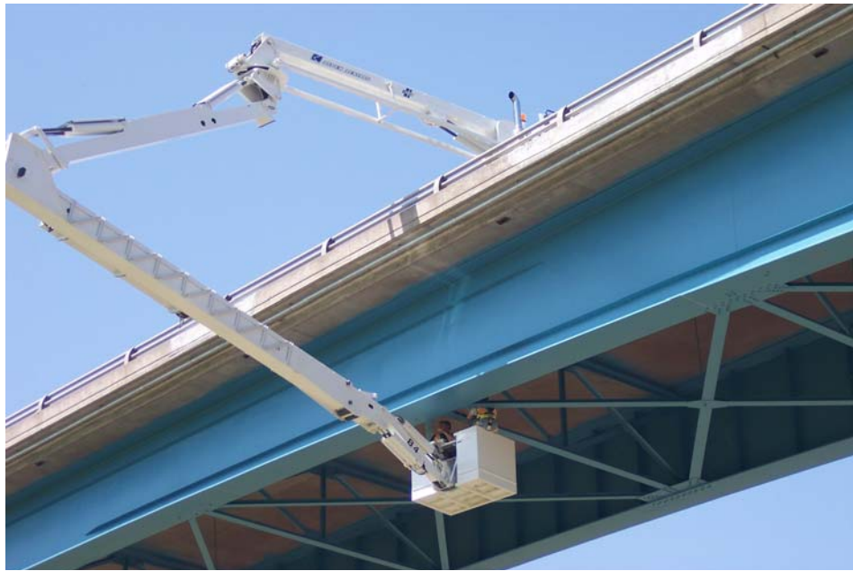
Figure 3-1: Snooper Used for Bridge Girder Access
