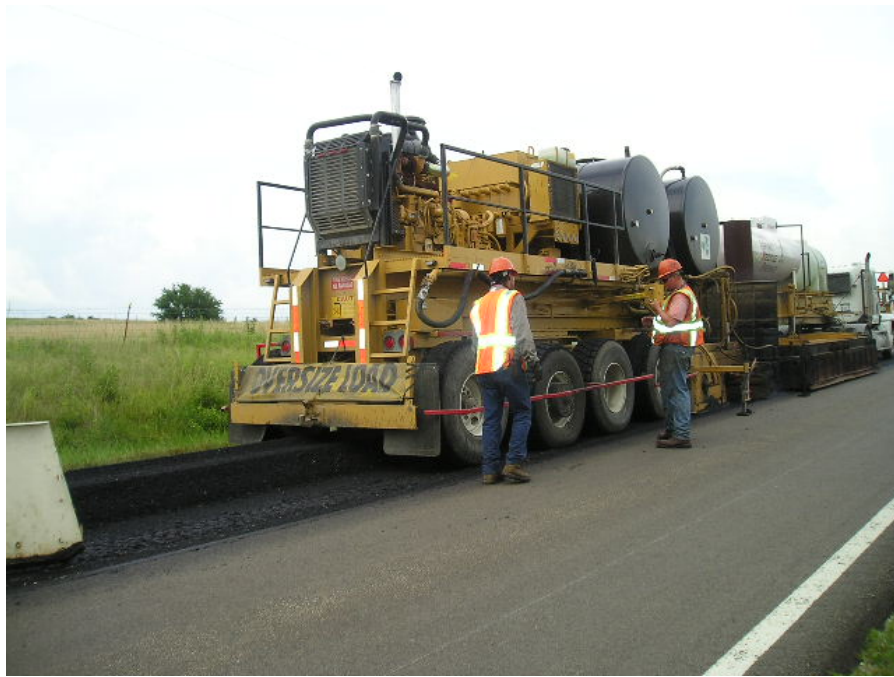
Fig. 32. Rejuvenating and mixing equipment
