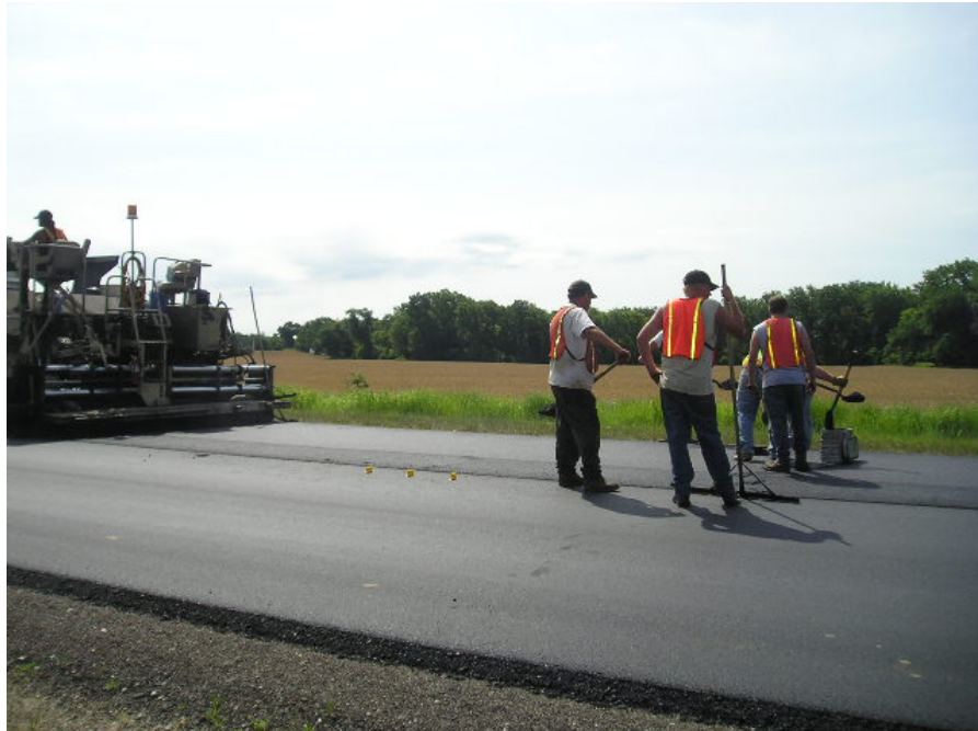
Fig. 26. Sampling the asphalt mix for lab test
