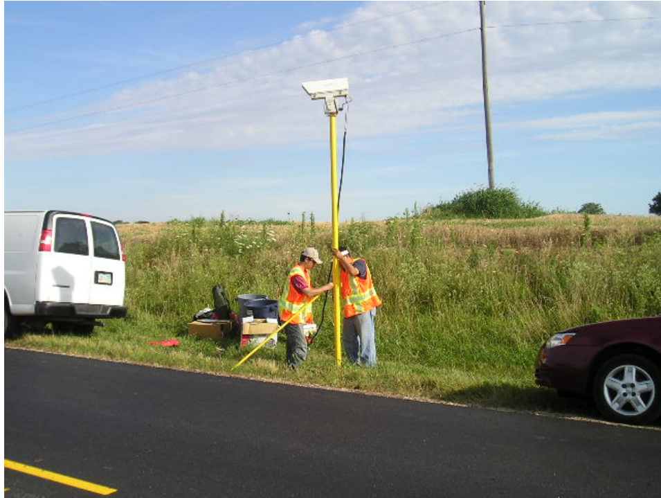
Fig. 15. Supporting the pole with three steel legs
