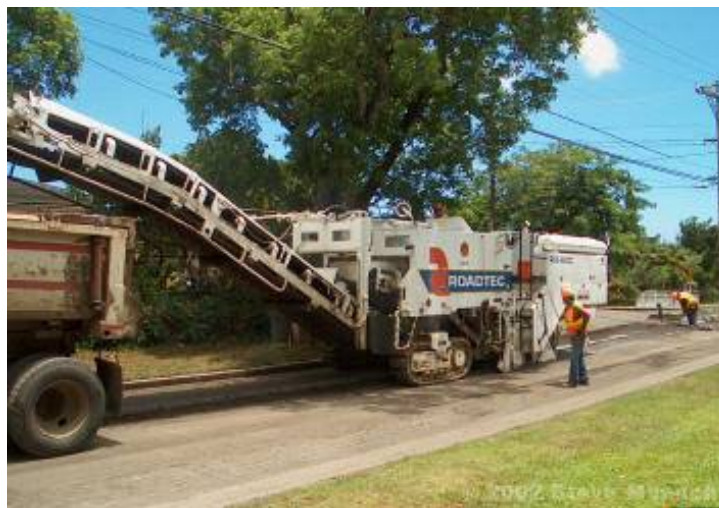
Fig. 23. Milling (Washington Asphalt Pavement Association 2002)
