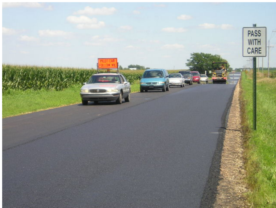
Fig. 22. Traffic control (single lane closure)
