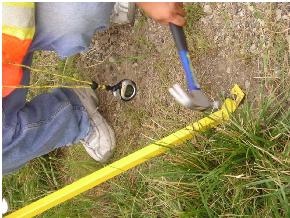
Fig. 16. Hammering big nails into the ground
