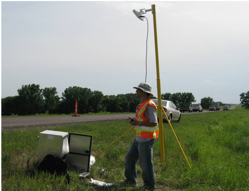
Figure 5.1: Installation of the speed detection device
