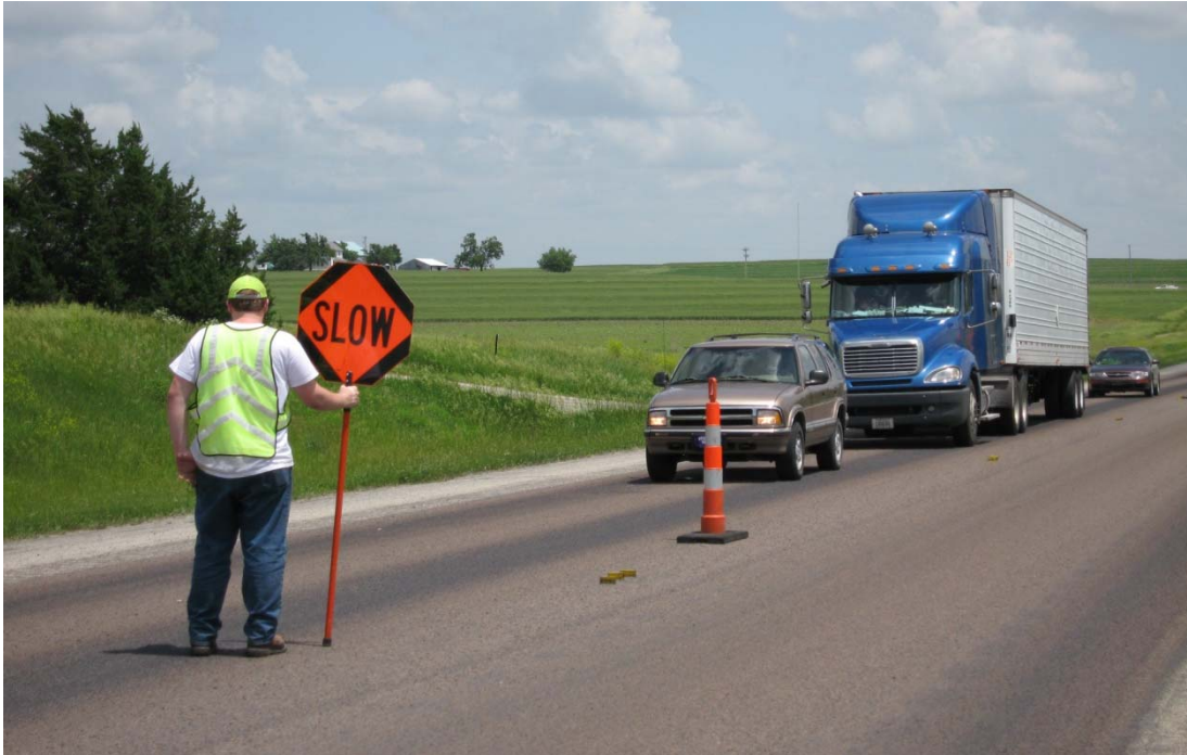
Figure 2.1: Flagger position in the work zone
