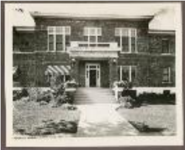
Figure 30: Administration Building, WIF, 1936 (Kansas Memory:229170).
