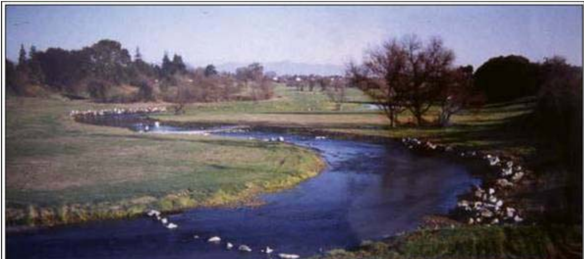
Figure 1: Rock Weirs Placed during the Restoration of Uvas Creek (Photo credit, Kondolf, et. al, 2001)
