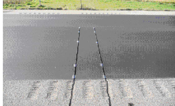
4. Completing the tube installation
