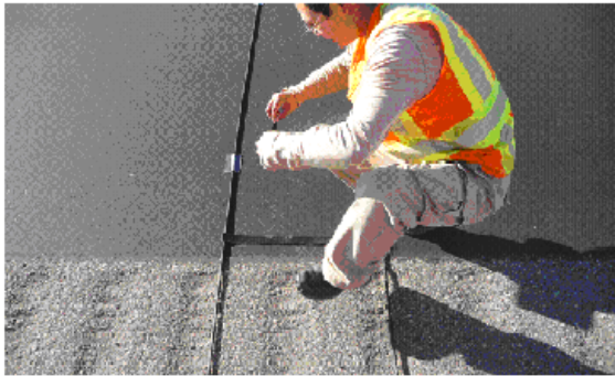
3. Installing tubes with a tape measure
